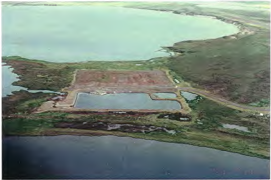
Figure 3. Aerial oblique of Inigok drilling site from southwest, showing the pad surrounded by lakes on three sides and the channel cut through the former flare pit (17 July 1991).
