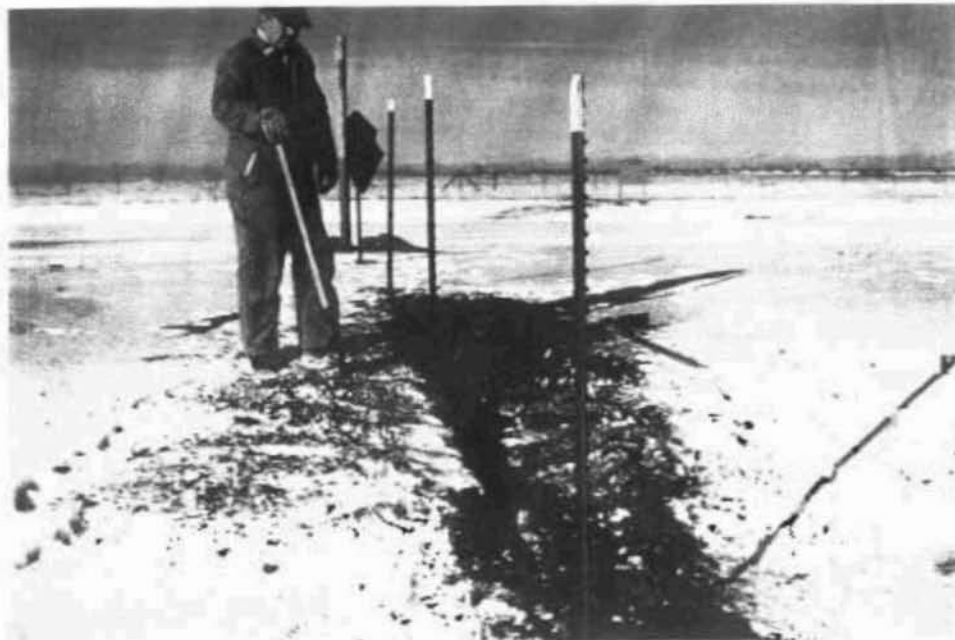
Figure 4. Installation of posts for a snow fence on Block 1 of the BP Put River No. 1 gravel pad experimental area (25 September 1990).
