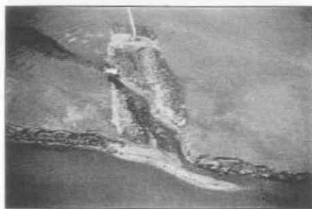
Figure 9. Aerial oblique views of Badami Pipeline on the west side of the Sagavanirktok crossing 22 July 1998 (upper) and 27 August 1999 (lower). Two sets of crawler tracks are prominent in the tundra to the left of the backfilled trench. A single faint set of tracks can be seen to the right of the pipeline above the helipad (upper photo). These marks are believed to have resulted from heavy equipment moving across the tundra during construction without protection from the ice pad. They may not cause thermokarst and will probably become vegetated naturally in time. Those in the margins of the Arctophila fulva bed are apt to persist as depressions in the soil for an indefinite period. Vegetation cover will obscure them more quickly in the wet habitats than on the dry sites. This type of tundra marking is relatively uncommon for the Badami Pipeline, and is pointed out here, because it appeared so obviously in these photos. Also important to note is the marked erosion and calving of the river bank that occurred between the 1998 and 1999 photos.
