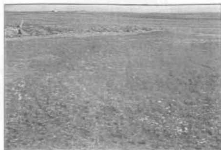
Figure 8. Northeastward from photopoint #2 at the west end of the Sagavanirktok river crossing. Left image shows backfill over the buried pipeline 14 August 1998, and the right view shows the same area on 27 August 1999 after water removed most of the backfill.
