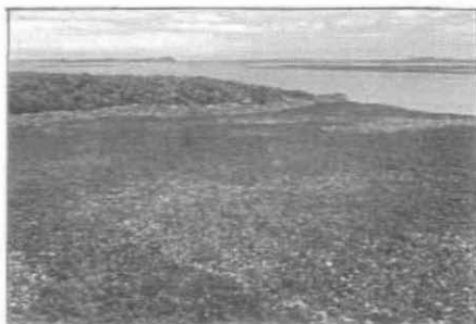
Figure 8. Northeastward from photopoint #2 at the west end of the Sagavanirktok river crossing. Left image shows backfill over the buried pipeline 14 August 1998, and the right view shows the same area on 27 August 1999 after water removed most of the backfill.
