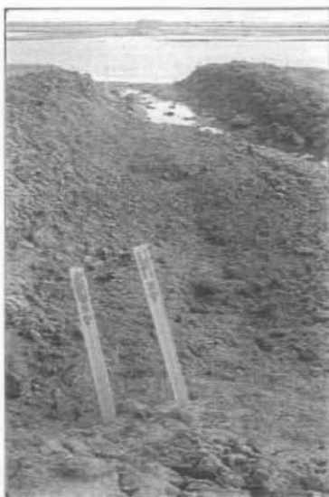
Figure 10. View eastward of backfilled trench over buried pipeline on the west side of the Sagavanirktok River. Photos were obtained, respectively on 14 August 1998 (left) and 27 August 1999 (right). Water was impounded in a subsidence over the pipeline in 1998, and had cut through the backfill during spring breakup in 1999. The east end of the river crossing can be seen in the distance.
