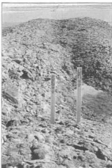
Figure 10. View eastward of backfilled trench over buried pipeline on the west side of the Sagavanirktok River. Photos were obtained, respectively on 14 August 1998 (left) and 27 August 1999 (right). Water was impounded in a subsidence over the pipeline in 1998, and had cut through the backfill during spring breakup in 1999. The east end of the river crossing can be seen in the distance.
