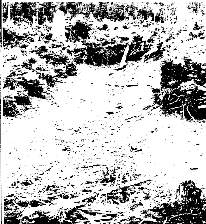
Figure 16.—Small landslip caused by road construction. Debris in foreground is lying on the road. Cut banks were about 6 or 7 feet high.
