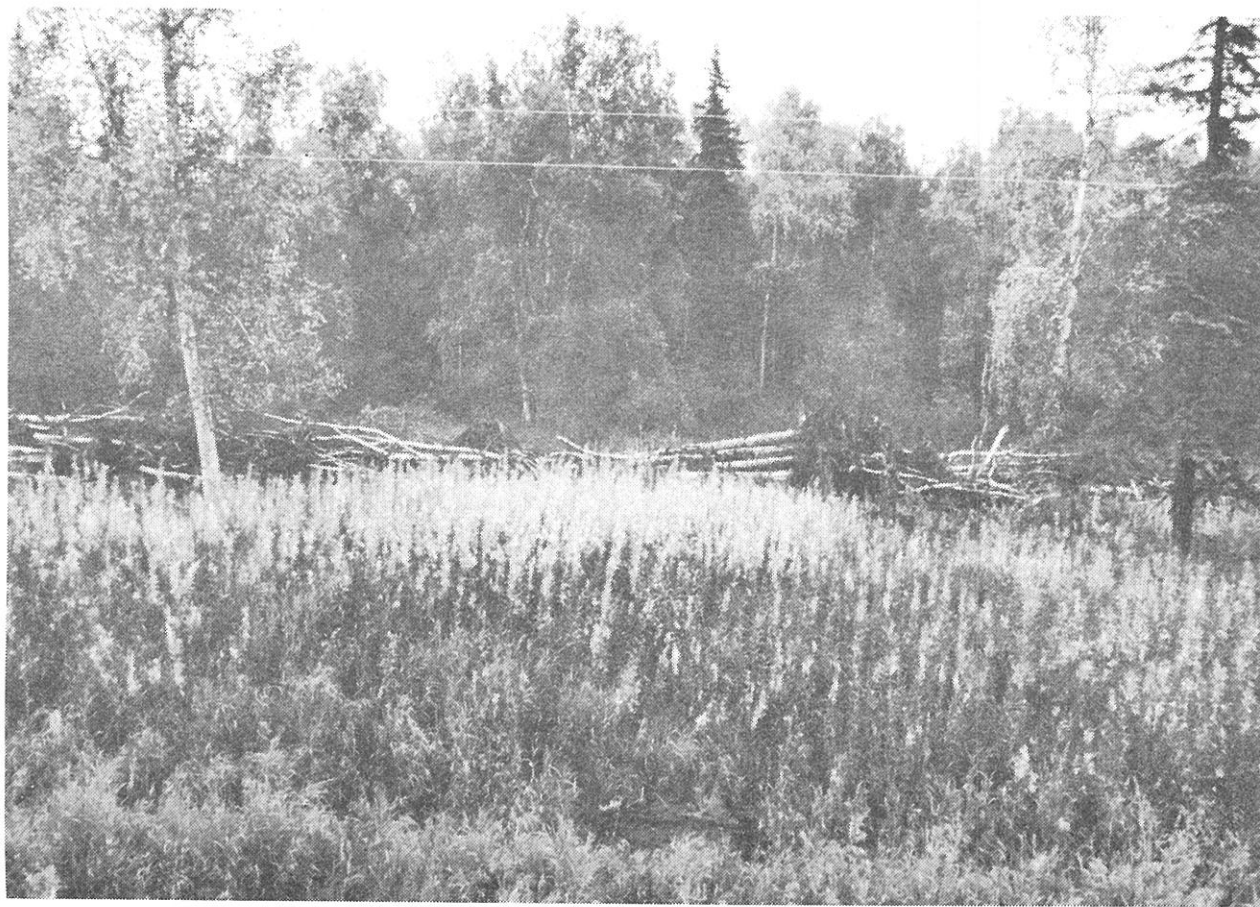
Clearing for Matanuska Electric Association (MEA) distribution line. Vegetation is predominantly poplar and spruce. Clearing was done by uprooting trees with a bulldozer.
