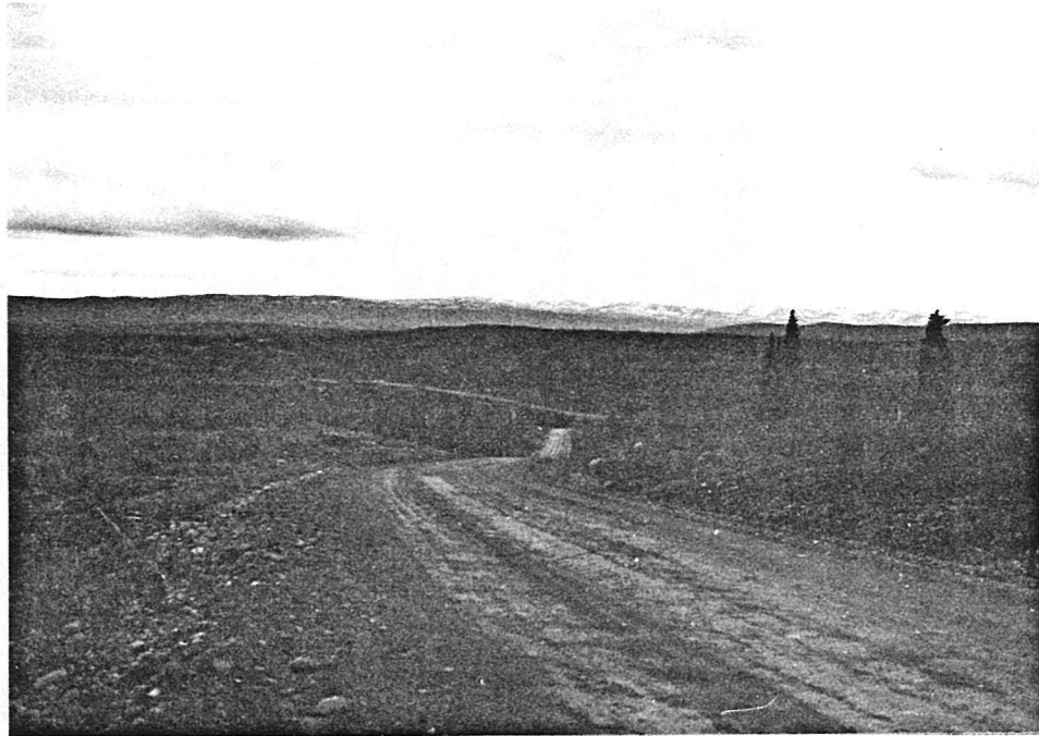
PHOTO E4.8.3: DENALI HIGHWAY (LOOKING SOUTHEAST) NEAR PROPOSED ACCESS ROAD JUNCTION. THIS IS A TYPICAL COMPACTED GRAVEL ROAD AND IS SIMILAR TO THE PROPOSED ACCESS ROAD
