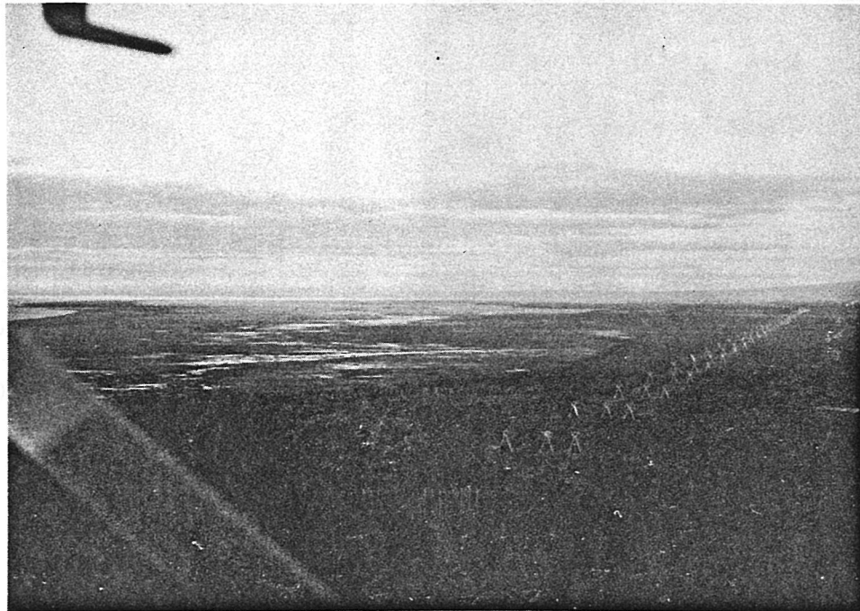
PHOTO E43.8.12: EXISTING TRANSMISSION LINES NORTH SIDE OF COOK INLET - SUSITNA RIVER LOWLANDS. THIS CORRIDOR IS SIMILAR IN SIZE AND TOWER DESIGN TO THE DEVIL CANYON TO GOLD CREEK CORRIDOR. NOTE THE STRAIGHT ALIGNMENT AND RIGID VEGETATION EDGES
