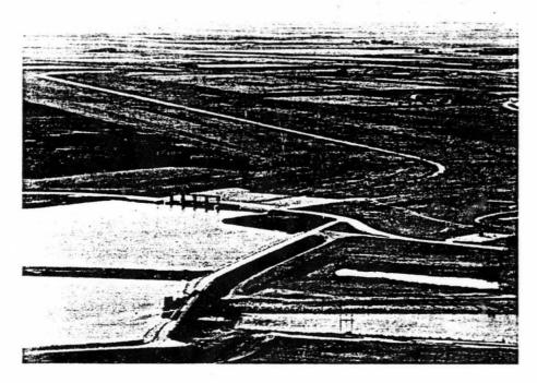
Diversion of water into the channel is accomplished by two control structures: a dam and spillway on the Assiniboine River, and a gated structure at the inlet to the diversion channel.
