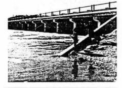
The Fairford River control is at the outlet of Lake Manitoba. This control structure permits effective regulation of Lake Manitoba water levels.
