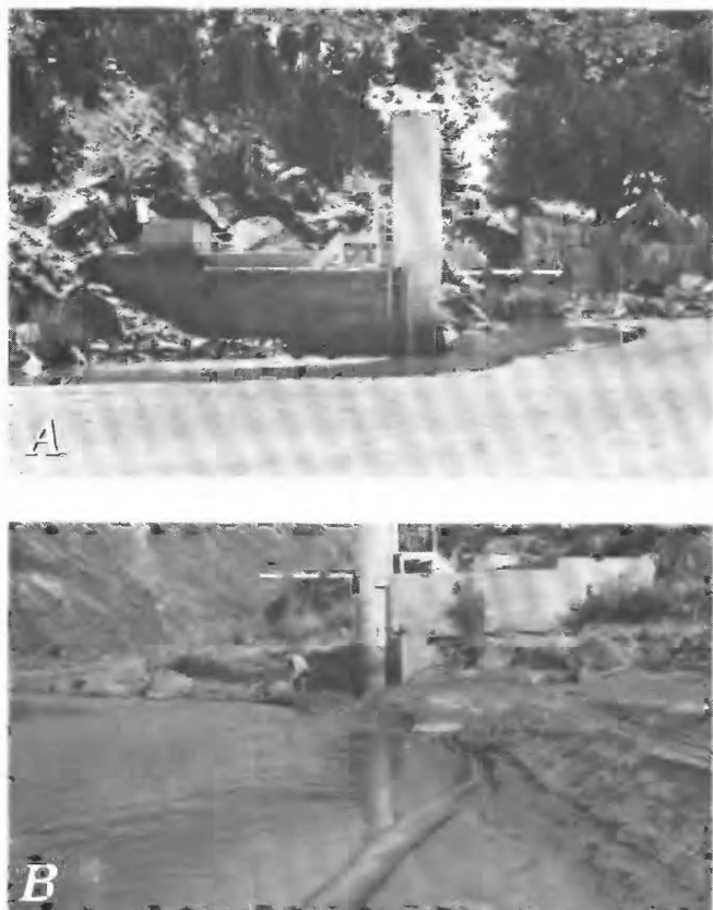
FIGURE 5.—Time progression of bed degradation and channel armoring at the streamflow-gaging station downstream from Jemez Canyon Dam, Jemez River, New Mexico. A, 1952; B, 1957; C and
