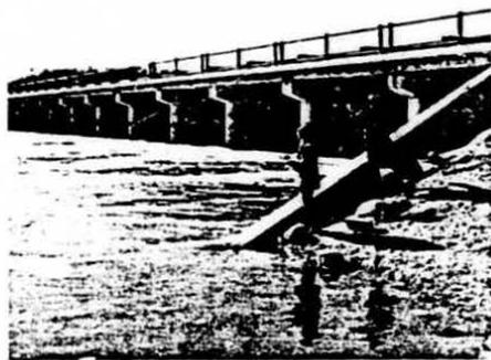
*The Fairford River control is at the outlet of Lake Manitoba. This control structure permits effective regulation of Lake Manitoba water levels.*
