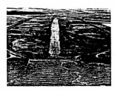
Concrete drop structures control erosion as the Diversion Channel drops between Portage la Prairie and Lake Manitoba.
