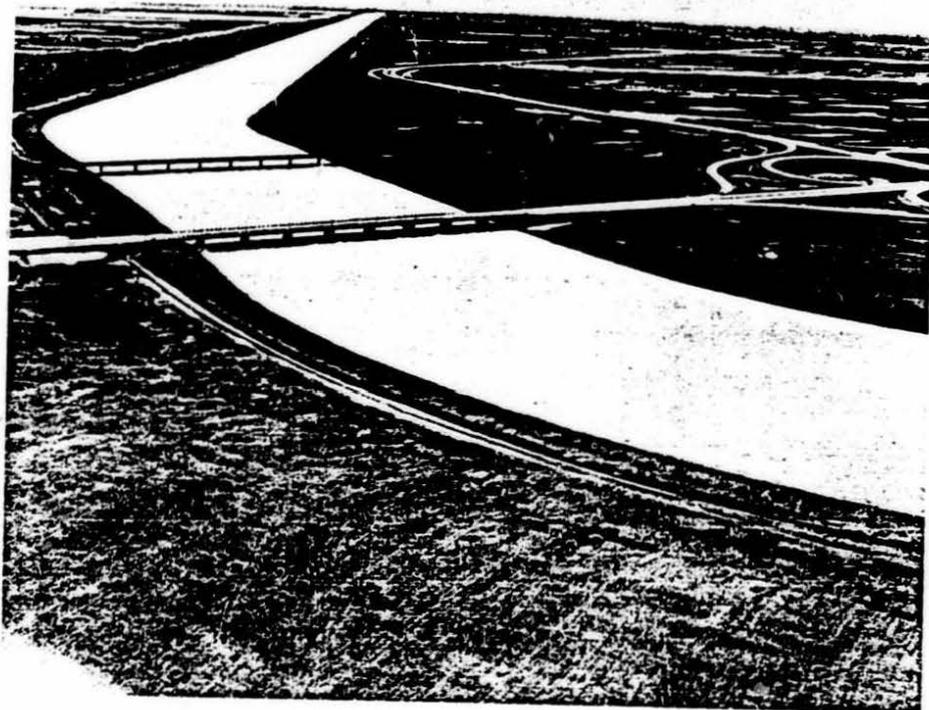
built south of Winnipeg to hold excess spring runoff, for slow release during the summer. These were not practical alternatives, however, as dredging the channel would have cost twice as much as a floodway, and a dam built south of Winnipeg creating a flood storage reservoir, would result in heavy flooding to farmland during flood conditions.
