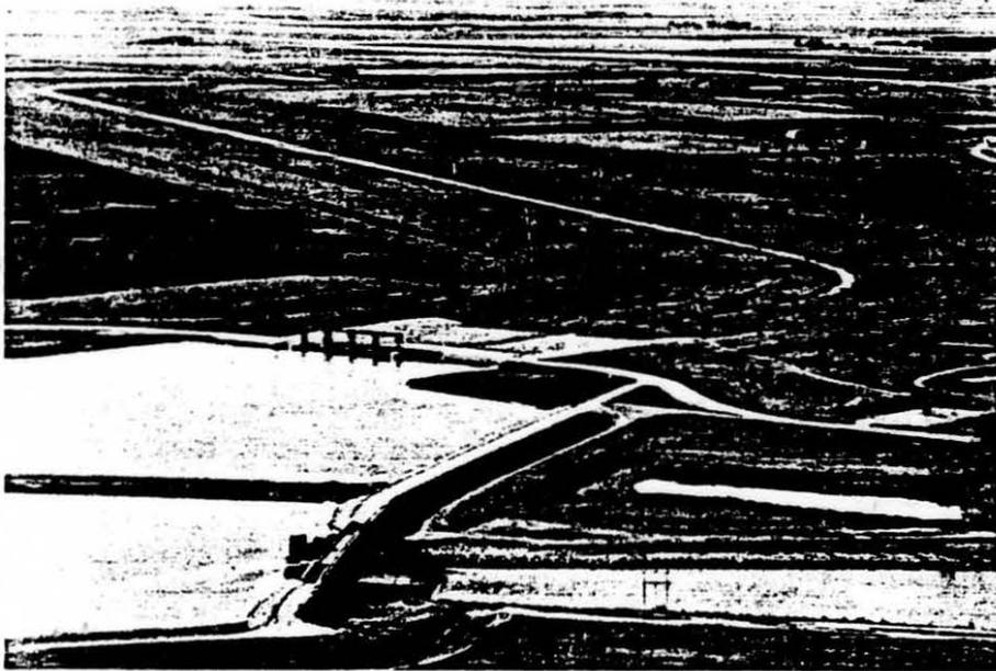
Diversion of water into the channel is accomplished by two control structures: a dam and spillway on the Assiniboine River, and a gated structure at the inlet to the diversion channel.
