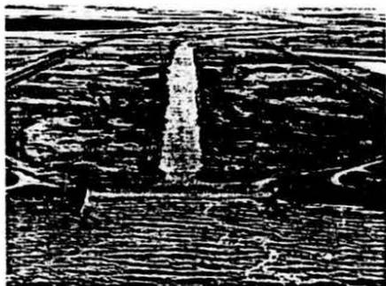
*Concrete drop structures control erosion as the Diversion Channel drops between Portage la Prairie and Lake Manitoba.*
