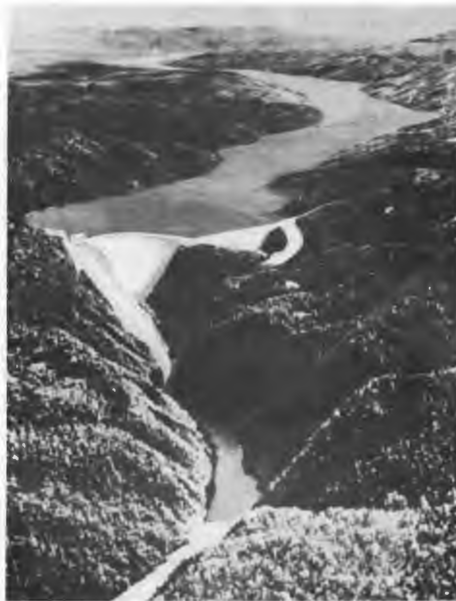
The Watana dam would be an earth-fill structure 885 feet high, 4 100 feet long, with an installed capacity of 1020 MW. The Devil Canyon dam would be a concrete arch dam 645 feet high, about 1500 feet long at the crest, with an installed capacity of 600 MW. The Watana dam would create a reservoir 48 miles long; Devil Canyon a reservoir 26 miles long.
