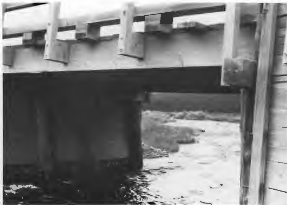
PHOTO 8.D.4 DENALI HIGHWAY BRIDGE. TYPICAL WOOD-FRAME STREAM CROSSING
