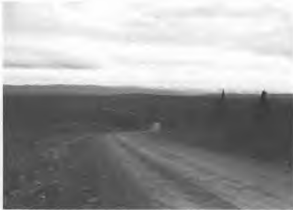
PHOTO 8.D.3 DENALI HIGHWAY (LOOKING SOUTHEAST) NEAR PROPOSED ACCESS ROAD JUNCTION. THIS IS A TYPICAL COMPACTED GRAVEL ROAD AND IS SIMILAR TO THE PROPOSED ACCESS ROAD
