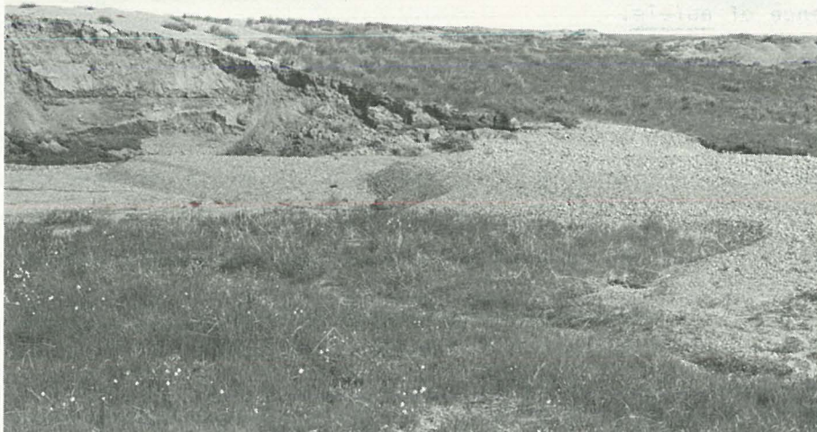
Figure 37. View of erosion of a diversion dam which acts as a long-term sediment source to Skeetercake Creek. Dunes in foreground are atypical of the undisturbed river.
