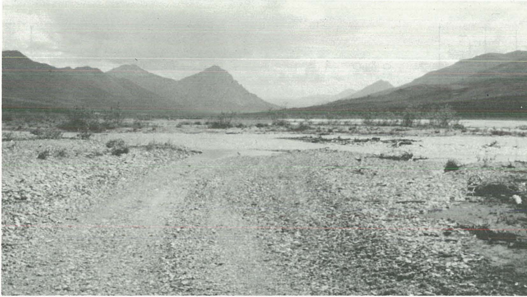
Figure 73. Compacted surface gravels in an access road leading to the Dietrich River-Downstream site.
