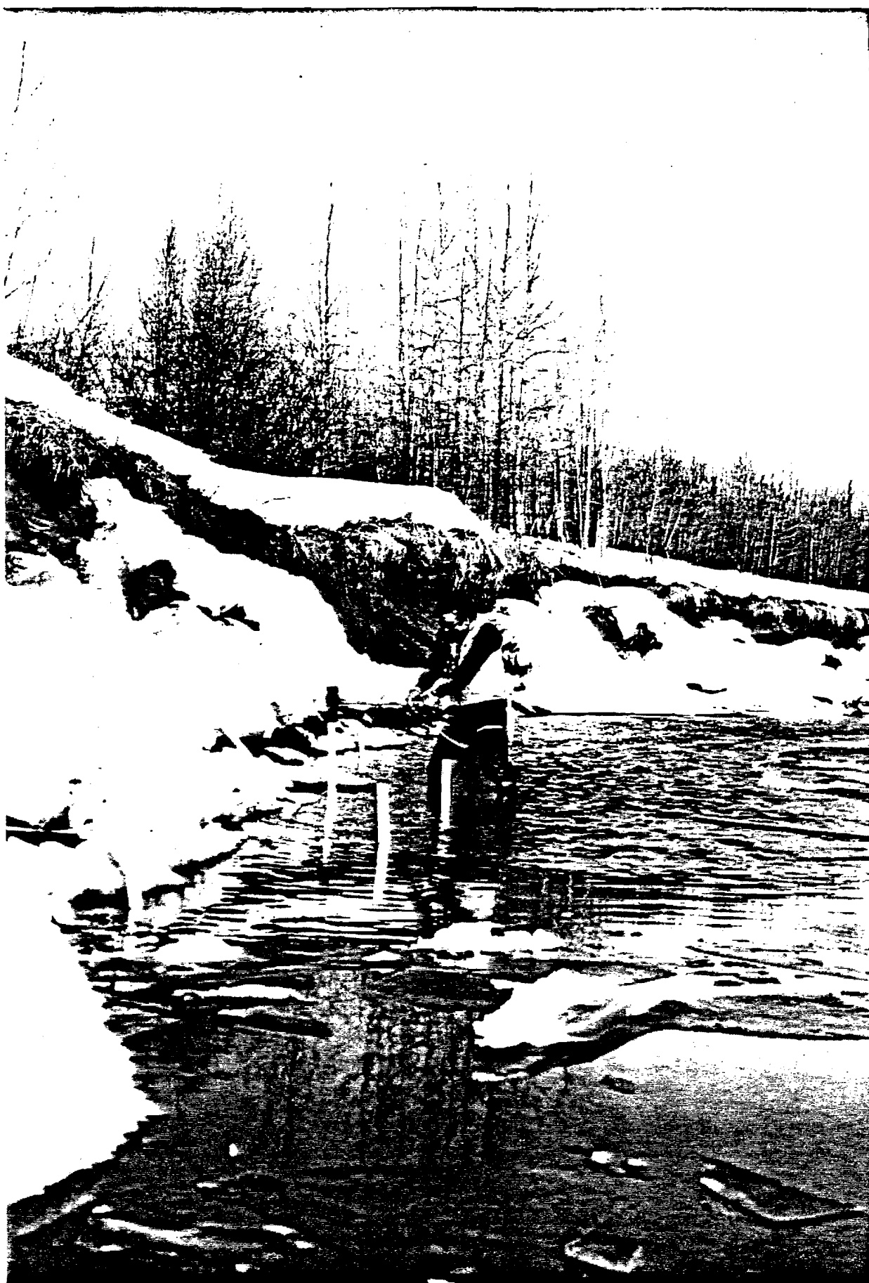
Plate 2. Installation of standpipes for monitoring intragravel water quality in Slough 11.
