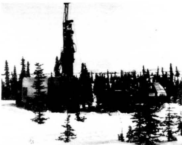
Drilling results help engineers design a more cost effective project. This Becker hammer drill tested over 50 locations at the Watana site.
