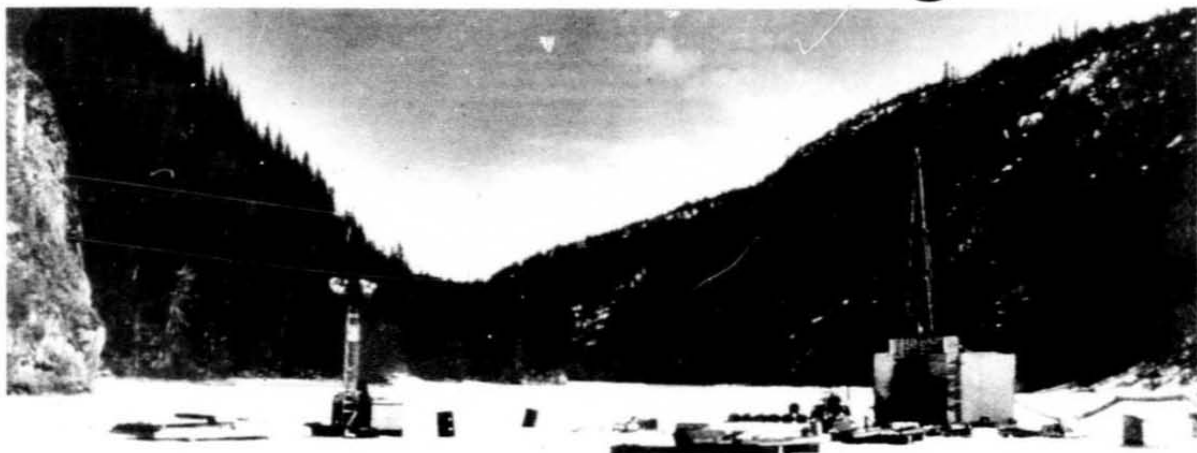
The winter geotechnical program used drilling and testing equipment on the river ice to confirm early work and improve design information.
