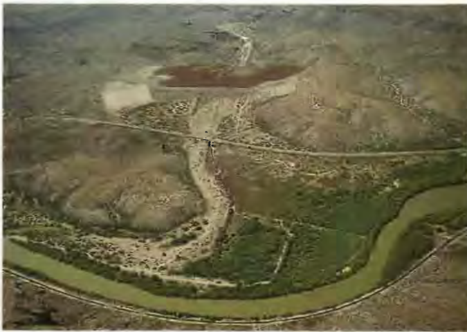
Broad Canyon Dam, a sediment-retention structure, upstream from the Rio Grande near Las Cruces, New Mexico
