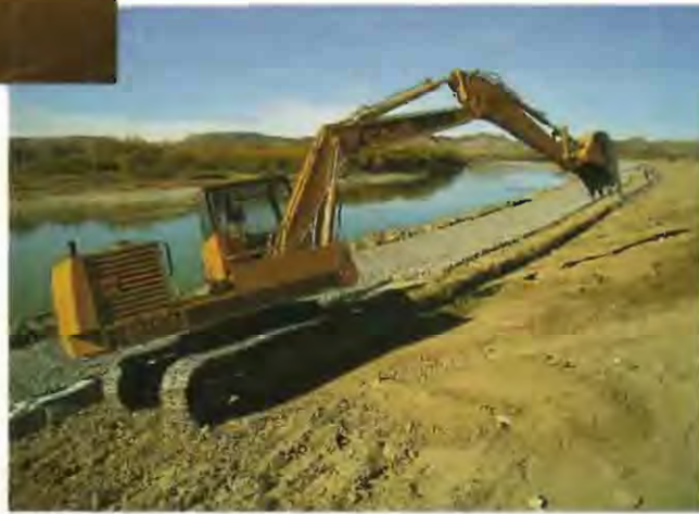
Dike reinforcement on the Rio Grande at Redford, Texas
