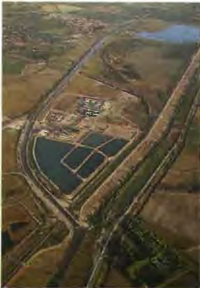
Riverside Dam on the Rio Grande downstream from El Paso, Texas
