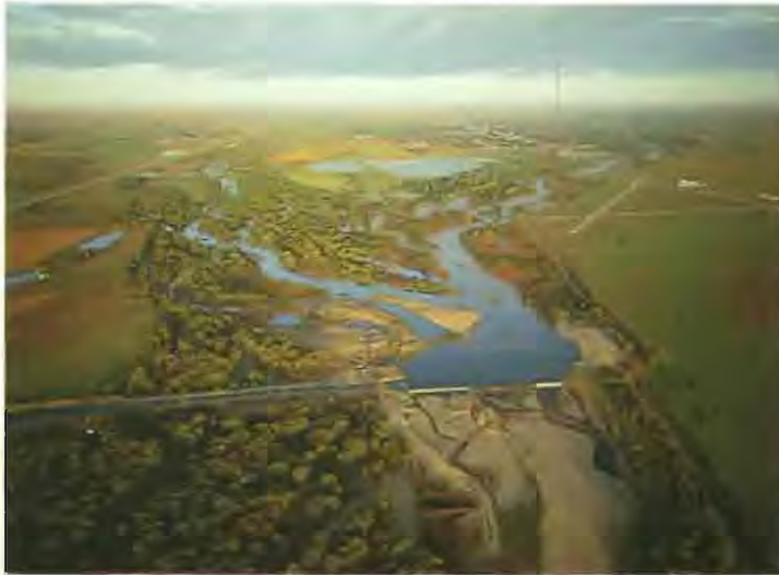
Diversion structure for the Tri-County Supply Canal below the confluence of the North and South Platte Rivers at North Platte, Nebraska.
