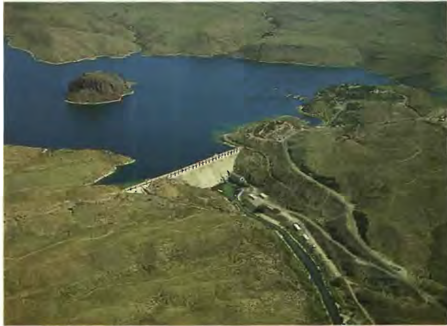
Elephant Butte Dam on the Rio Grande at Truth or Conse- quences, New Mexico
