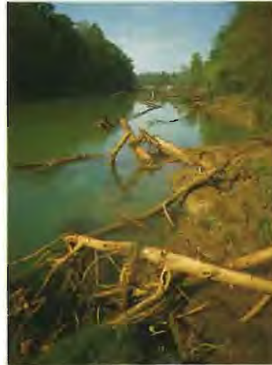
Eroded banks 2 miles below Buford Dam
