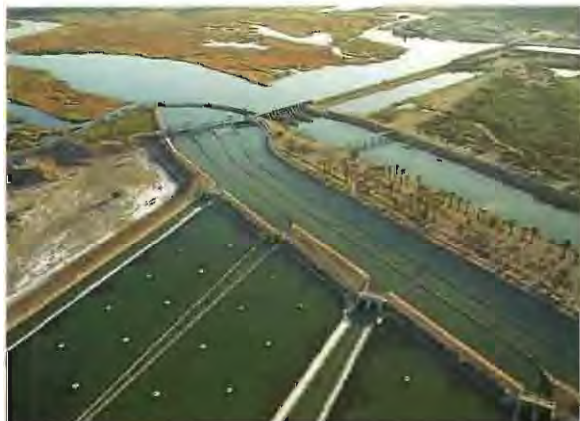
Imperial Dam north of Yuma, Arizona
