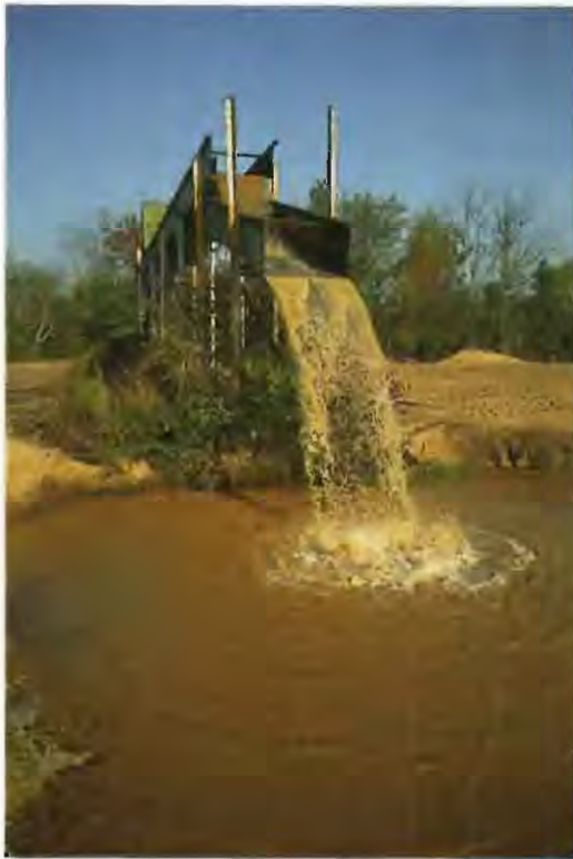
Dredging operation on the Chattahoochee River in Duluth, Georgia
