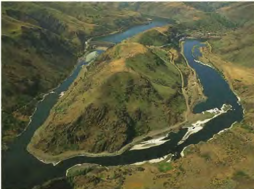
Oxbow Dam, part of the Hells Canyon Complex, on the Snake River, Idaho
