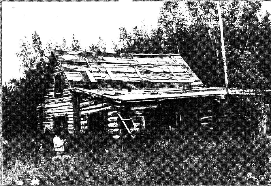
4. Bob Arnold's Road House Arnold is buried nearby but exact loc'n is not known. Floor is falling in — a new roof would save from further deteriorization.
