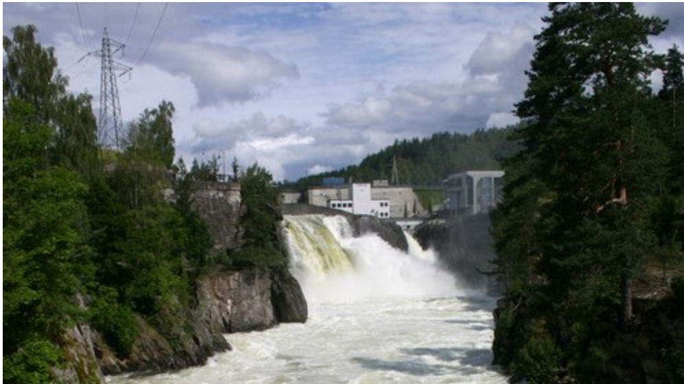
Figure 5-1. Tinnelva Hydropower Plant (Photo: Ånund Killingtveit, from http://www.forskningsradet.no ).
