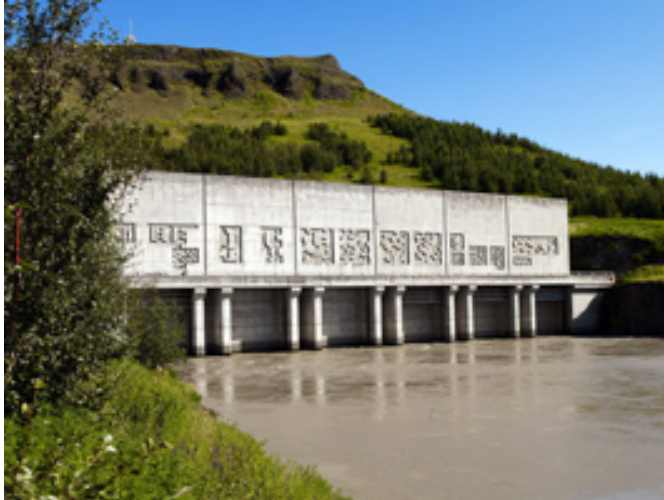
Figure 5-2. Burfell Hydropower Project on Thjorsa River, Iceland (photo from http://www.hydroworld.com ).
