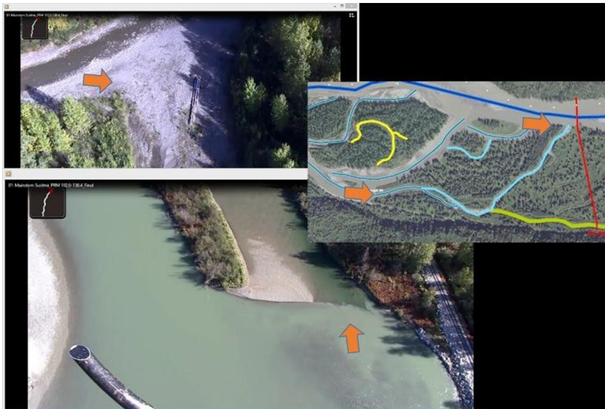
Figure 10. Channel if FA 128 classified as a side channel. However, the conditions at the upstream end of the channel and clear water are the same as the channels in FA 104 and FA 113 which were classified as side sloughs. Characteristics are consistent with side slough and not side channel classification.
