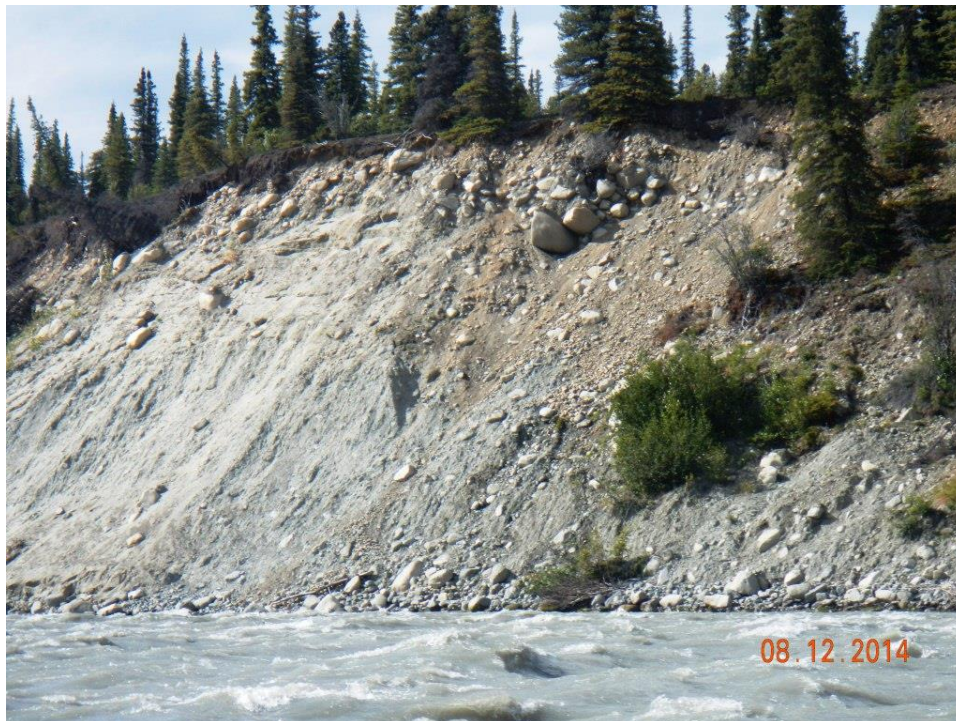
Figure A.2-38– High eroding lateral moraine with large cobbles and boulders at PRM 235 (P714).
