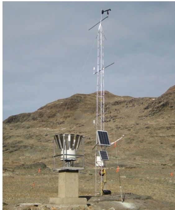
Figure 2. Example Meteorological Station Installation
