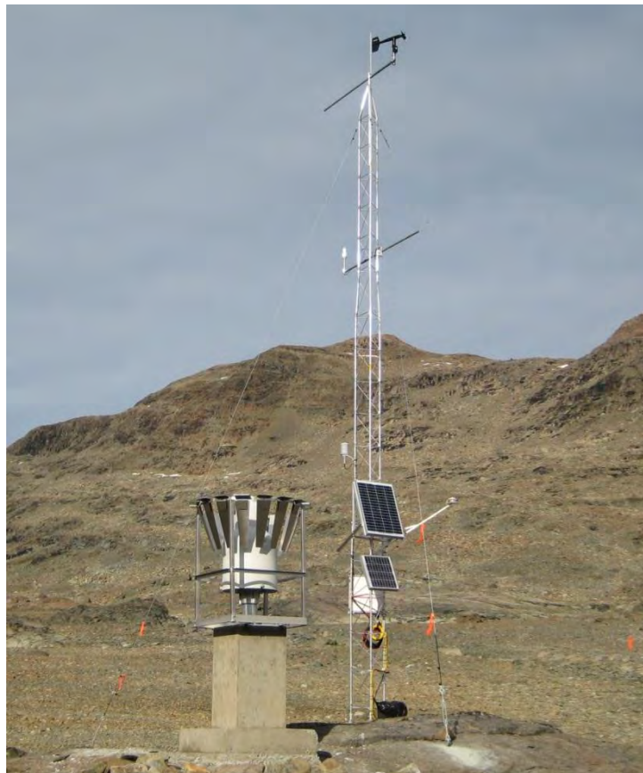
Figure 3. Example Meteorological Station Installation
