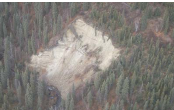
Figure 4-1. Sloughing soils in the South Rail alignment
