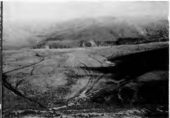
Fig. 5. (left) Access road--ground view. This road was constructed with a dozer. Surface vegetation and thawed soil were removed so wheeled vehicles could be driven over the frozen ground. It is about 3 feet deep at this place and about 1/4-mile long. Fig. 6. (right) Access roads--aerial view. These ATV trails have been used for years for mining claim access in the Kantishna area. Several miners use these trails with tracked vehicles or other types of ATV's. Some of the trails have revegetated naturally over the years. The trails are on d-2 lands in the proposed Mount McKinley National Park expansion.
