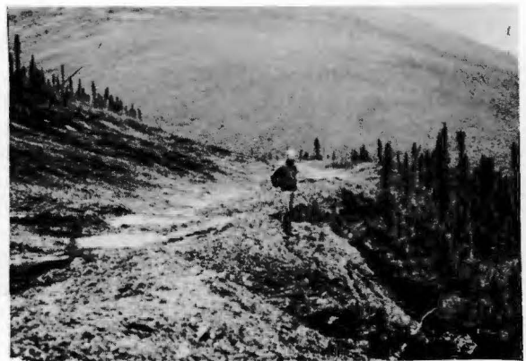
Fig. 1. (left) Water ditch--aerial view. The ditch was constructed in June 1974 by a miner to bring water to his claims. It has not been used. Located on d-1 lands near Eagle Summit on the Steese Highway, it is about 3 miles long. Fig. 2. (right) Water ditch--ground view. The miner constructed the ditch by bulldozing surface vegetation and mineral soil downhill to form a berm. The disturbed area is about 150 feet wide. Several breaks have occurred from normal surface runoff.
