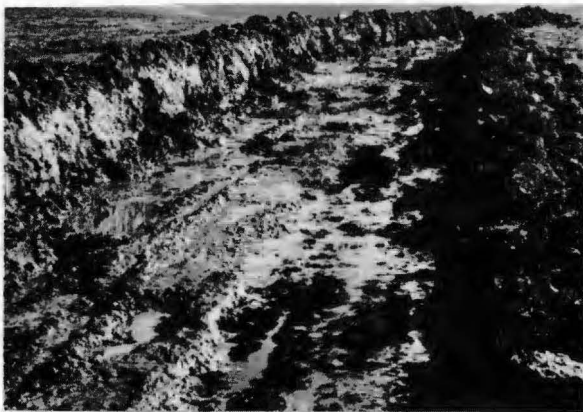
Fig. 5. (left) Access road--ground view. This road was constructed with a dozer. Surface vegetation and thawed soil were removed so wheeled vehicles could be driven over the frozen ground. It is about 3 feet deep at this place and about 1/4-mile long. Fig. 6. (right) Access roads--aerial view. These ATV trails have been used for years for mining claim access in the Kantishna area. Several miners use these trails with tracked vehicles or other types of ATV's. Some of the trails have revegetated naturally over the years. The trails are on d-2 lands in the proposed Mount McKinley National Park expansion.
