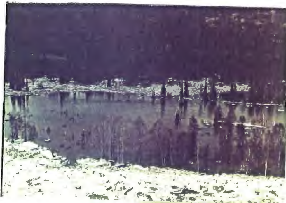
FIGURE 5.6 FLOODED TRACKS AND OVERBANK CAUSED BY ICE JAM AT CRX-11 MAY 13, 1982 PHOTOGRAPHY COURTESY OF THE ALASKA RAILROAD
