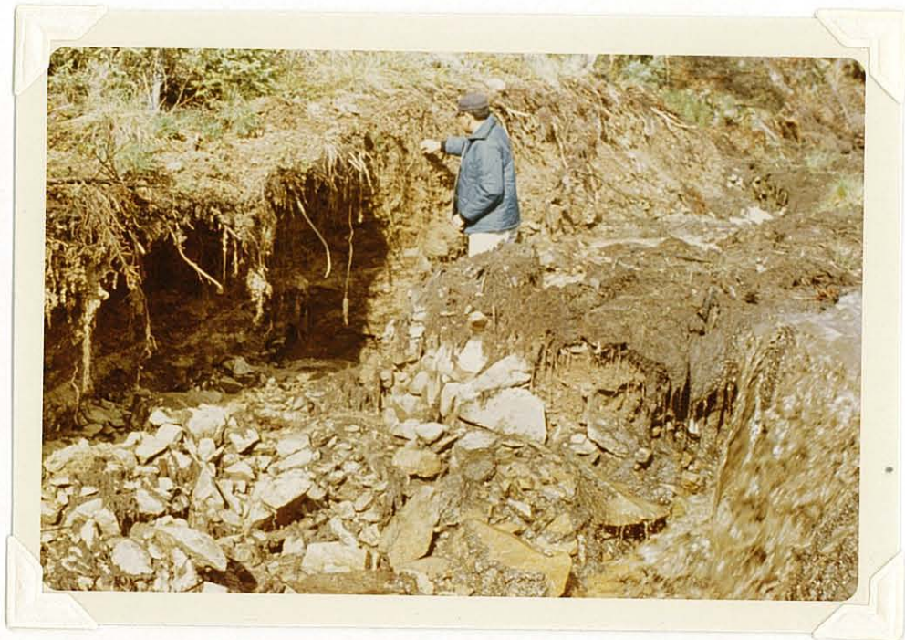
Photo No. 7 - Shows a well drained soil on south slope -- Y-34 Fire area. Fire line constructed in drainage bottom adjacent to slope has eroded down to bedrock.
