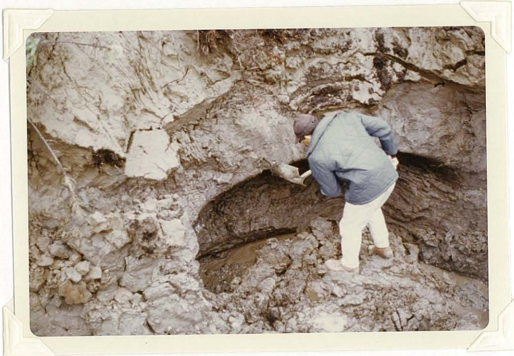
Photo No. 2 - Deep gully (approx. 10') on Goldstream Fire showing melting ice lenses and permafrost.
