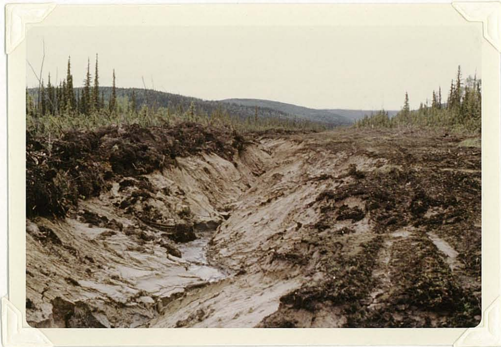
Photo No. 1 - Dozer-constructed fire line on Goldstream Fire showing debris berm in left center, gully in center, and unvegetated cleared line to right.
