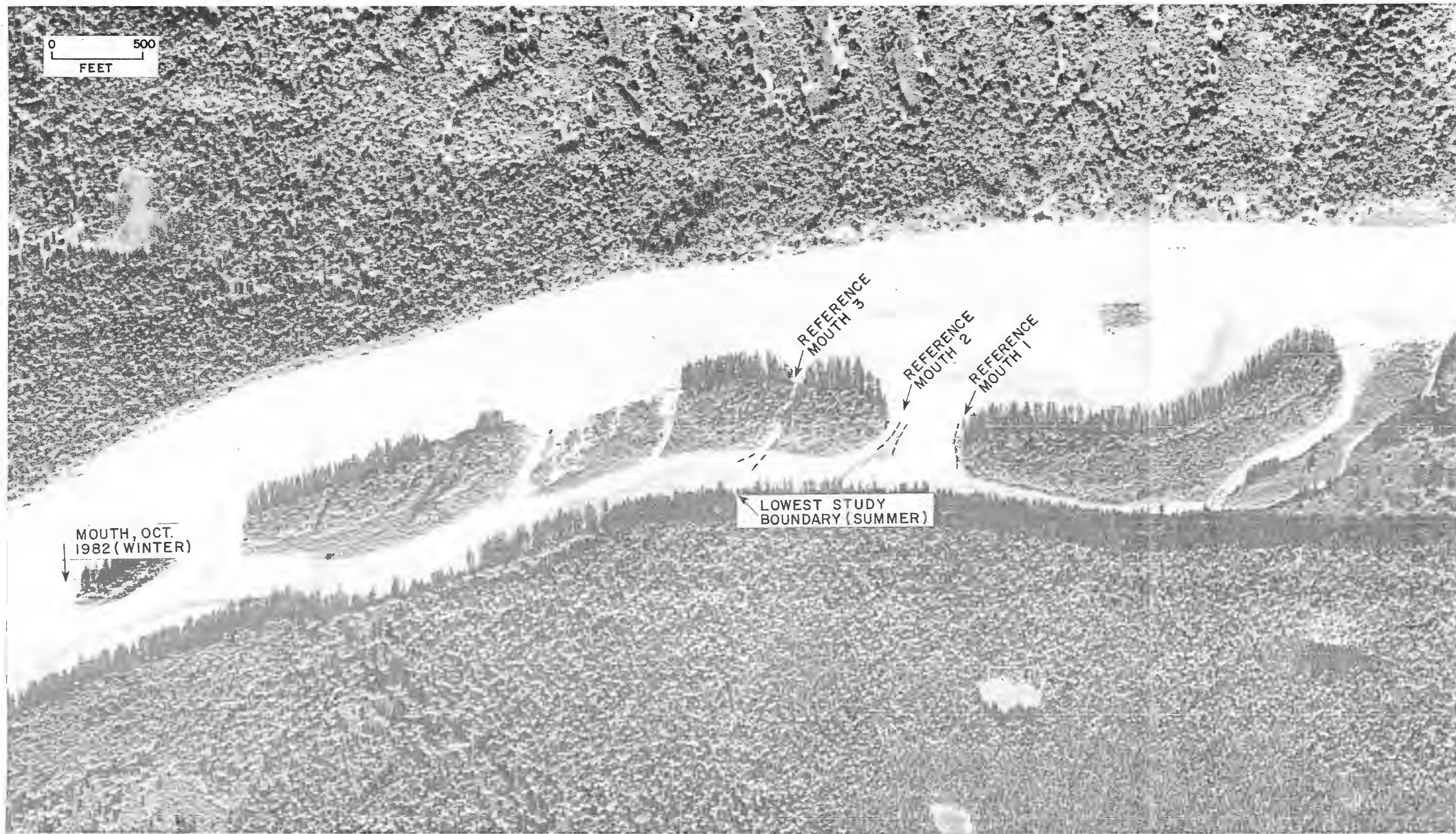
Appendix Plate 4-F-17. August 1980 aerial photograph of Slough 21 (RM 142.0). The Susitna River flows from right to left in this photo.
