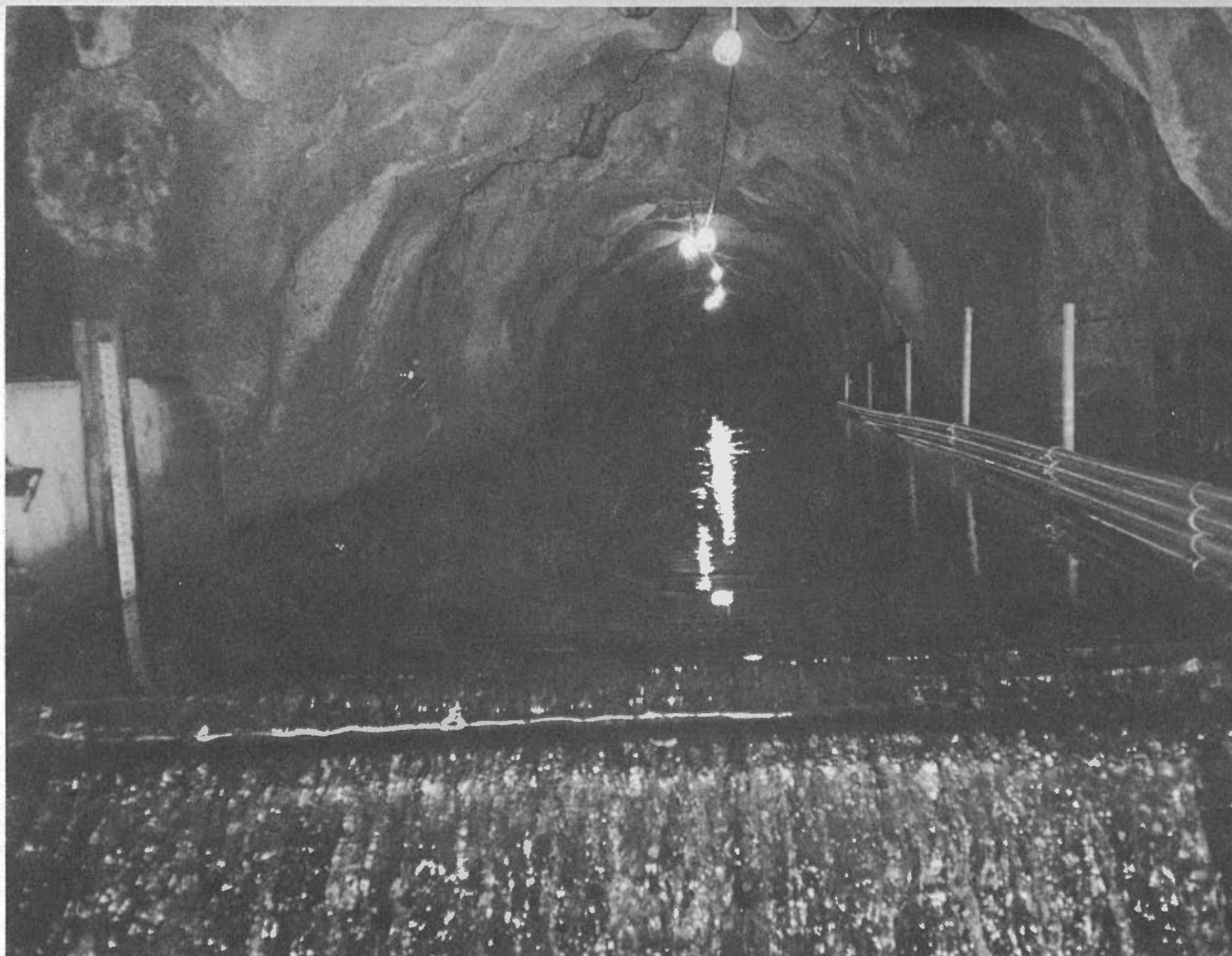
Figure 17-4. Twin Falls juvenile fish screen, downstream end of 136-foot-long left-side screen.
