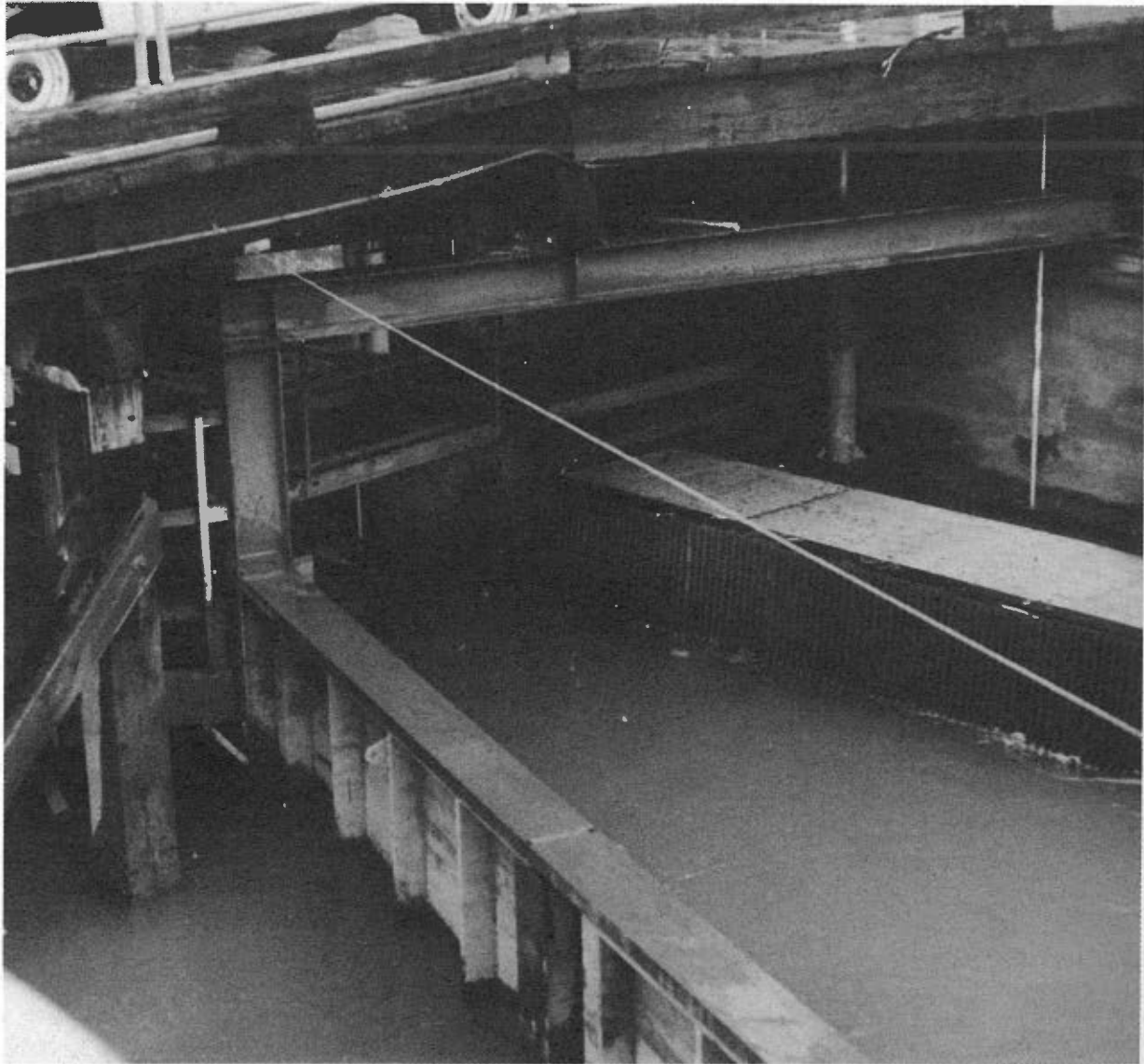
Figure 16-8. Training wall used to guide migrants to T. W. Sullivan Unit 13. The Unit 13 intake is under the bridge. The intakes for Units 1 through 12 are to the right of the bridge, through the bar racks.
