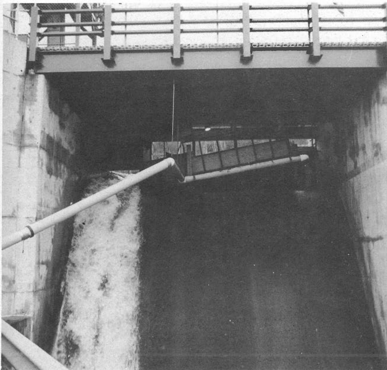
Figure 12-9. Fish sluice adjacent to the Little Falls powerhouse. A temporary fish evaluator is in the sluiceway.
