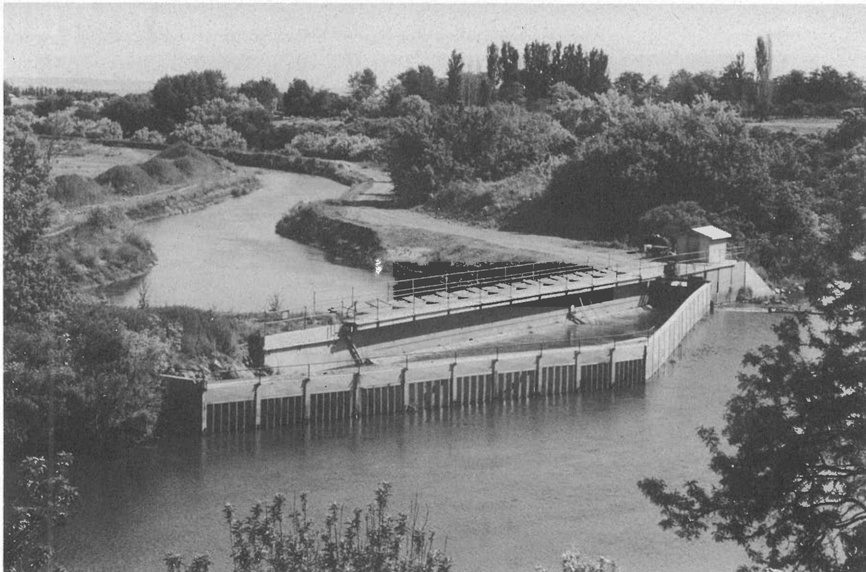
Figure 9-3. Jim Boyd trash racks, training wall and fish screen support structure.
