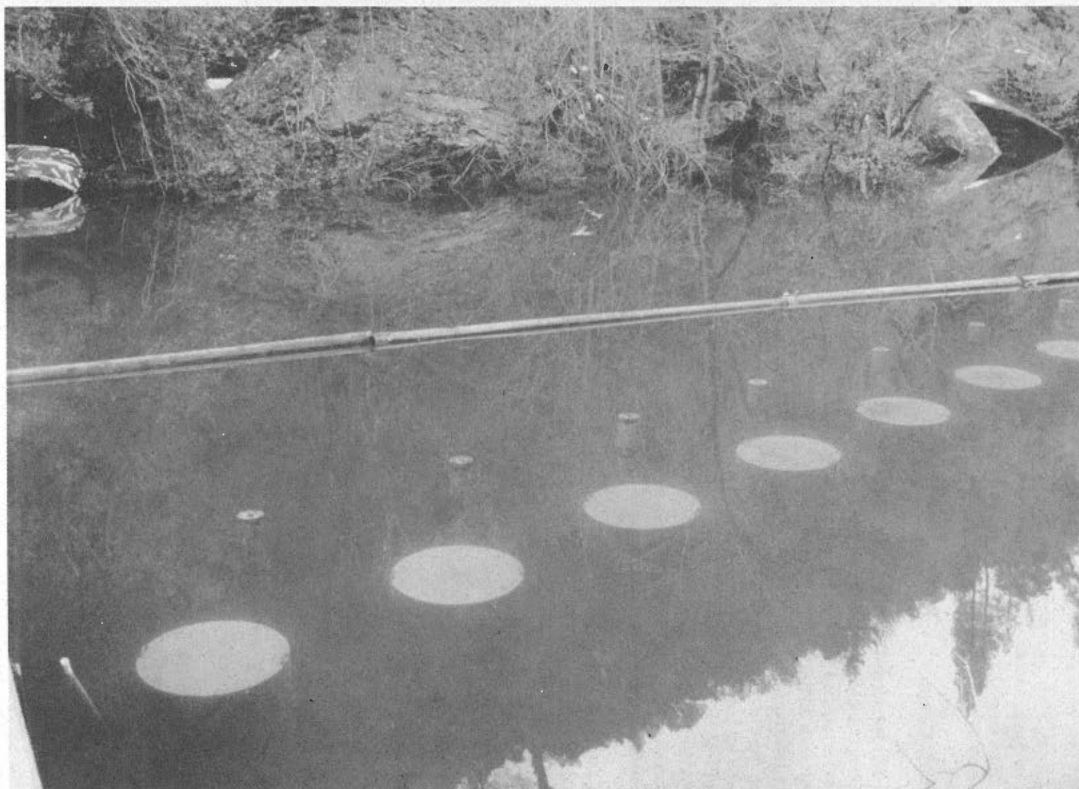
Figure 5-12. Arbuckle Mountain cylindrical wedge wire screens under water.
