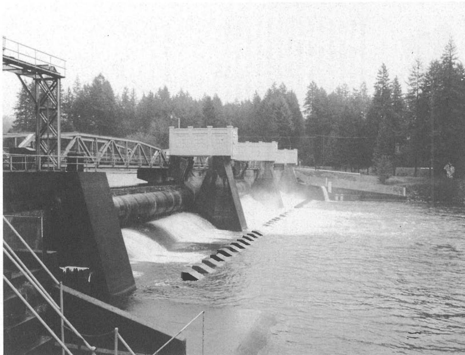
Figure 11-2. Leaburg diversion dam, viewed from the right bank. Left-bank spill is for left-bank fish ladder attraction flows.
