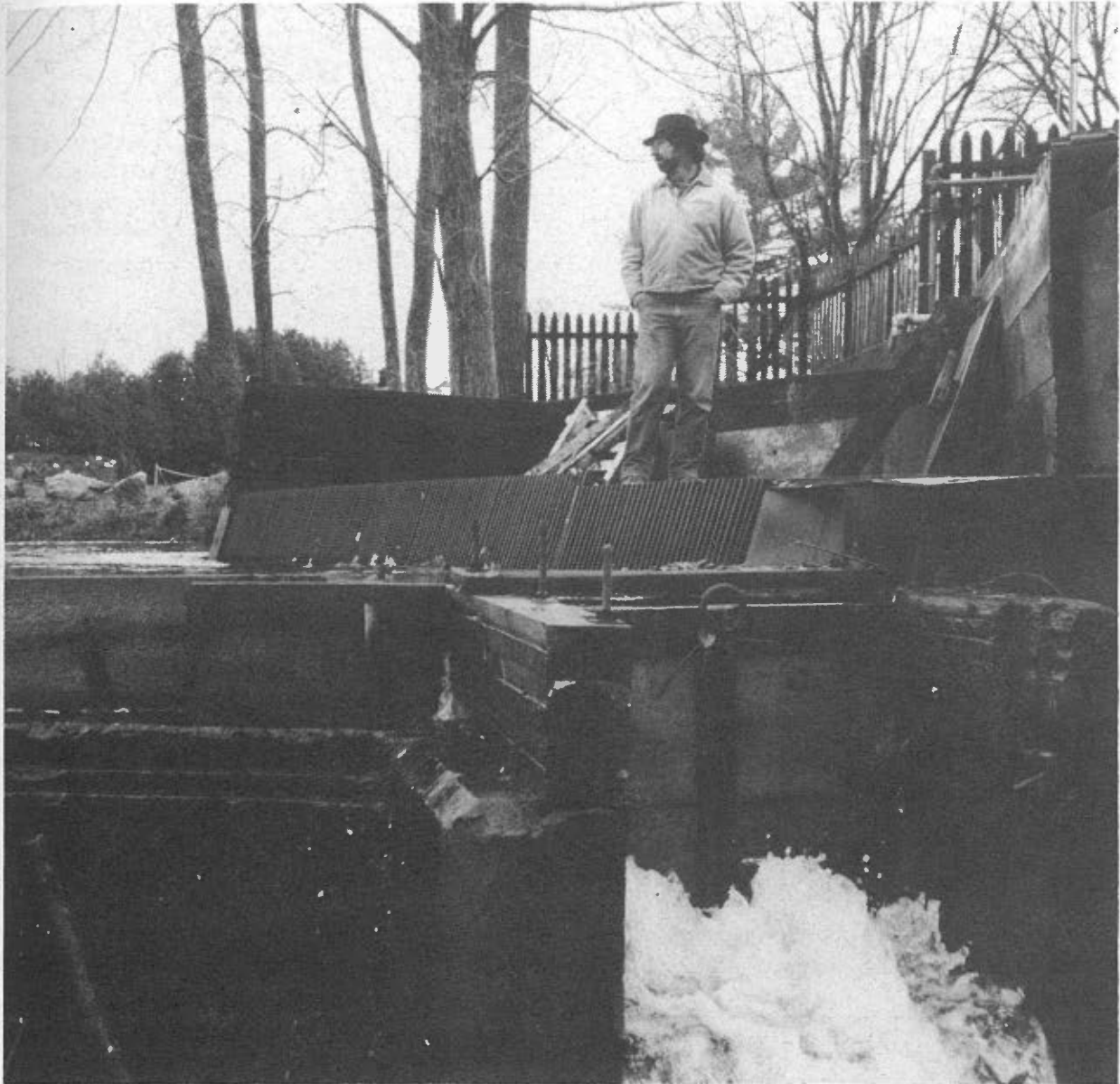
Figure 18-5. Wadhams project diversion dam, angled bar racks, and bypass used seasonally with wood deck sluiceway.
