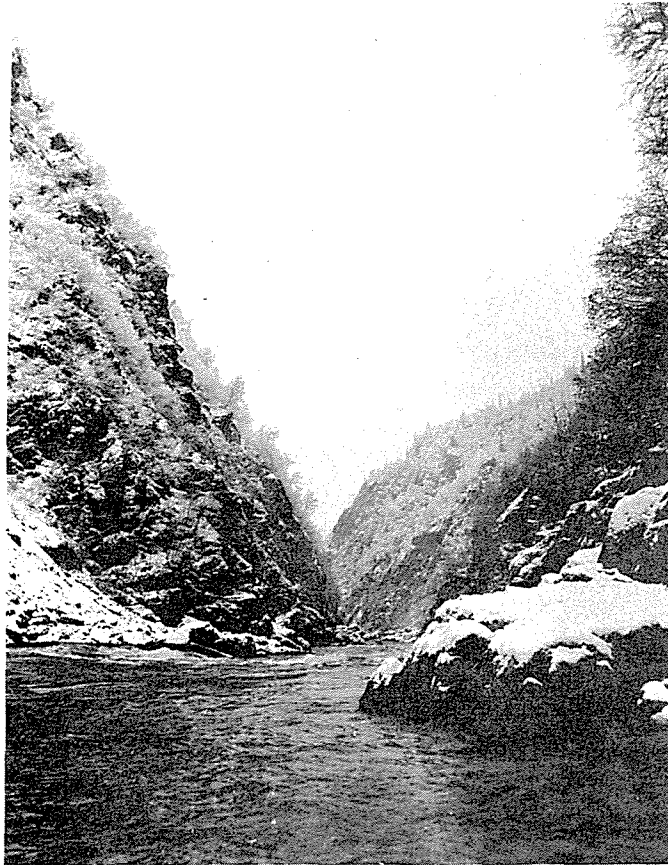
U. S. B. R. Photo Figure 3. View of proposed Devil Canyon Damsite, showing rapids and river gorge.
