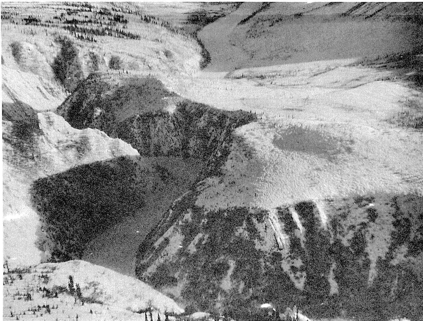
View of Vee Canyon damsite. (looking upstream)
