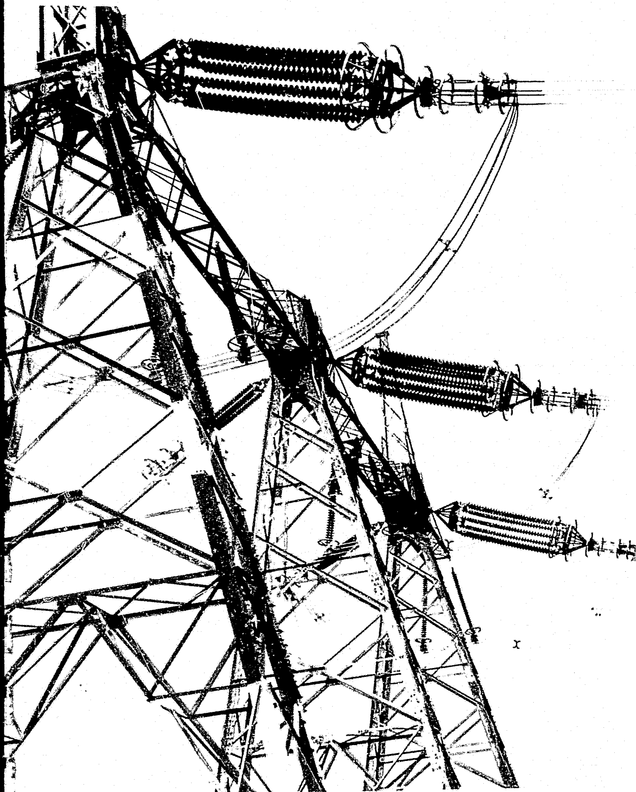
Jumper arrangement for the South Bank towers, river crossing line 1
