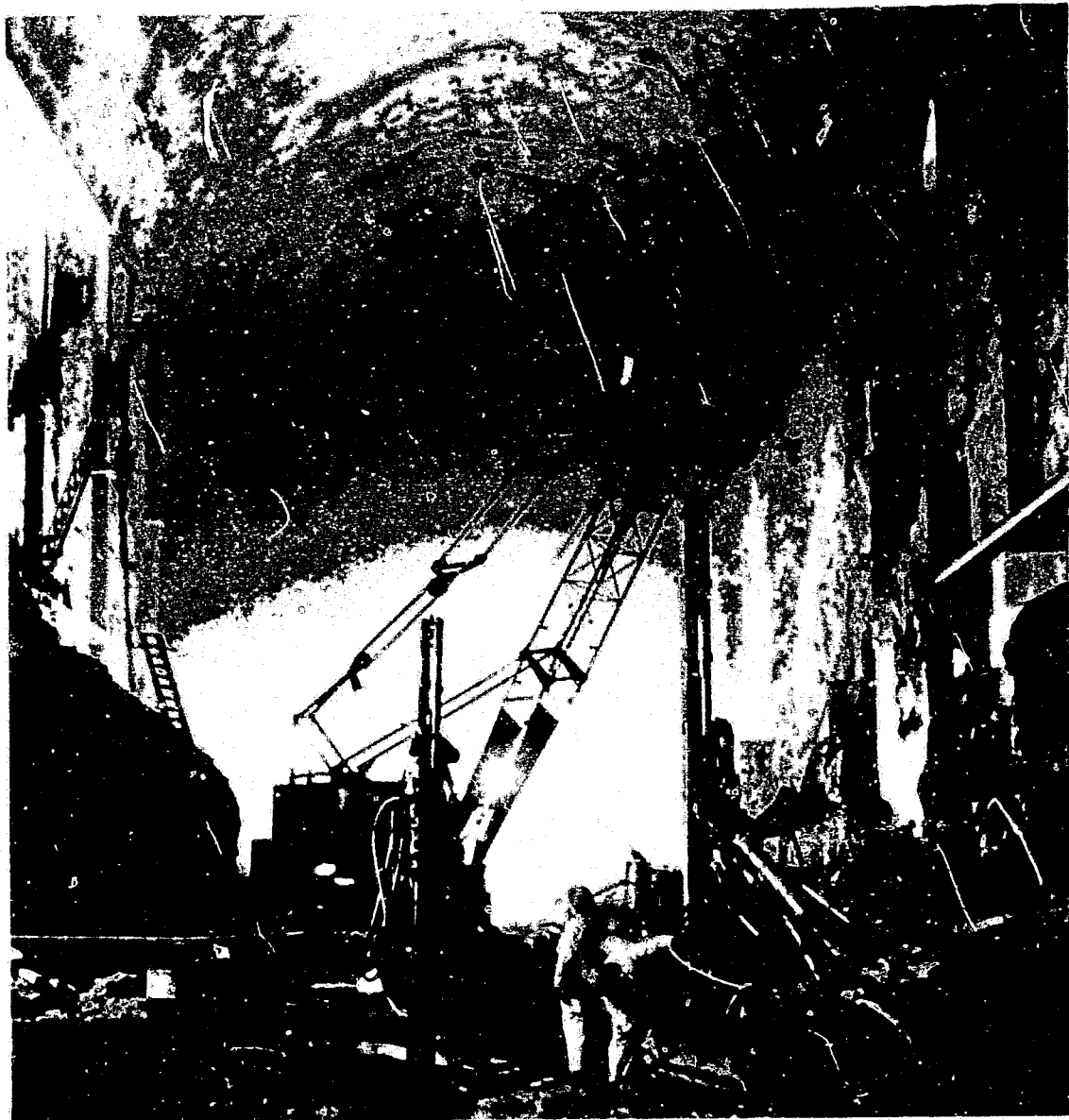
Excavation of the tailrace surge chamber
