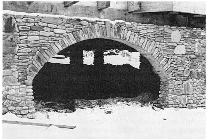
Winter in Alaska (left) often slows construction. The unique stone arch is constructed of river rock (above).
