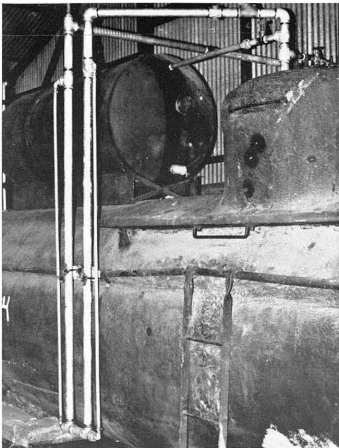
Methane originators (previous page). A gas collection dome (left) sits atop the digester. (above) McKee stands next to the insulated digester tank.
