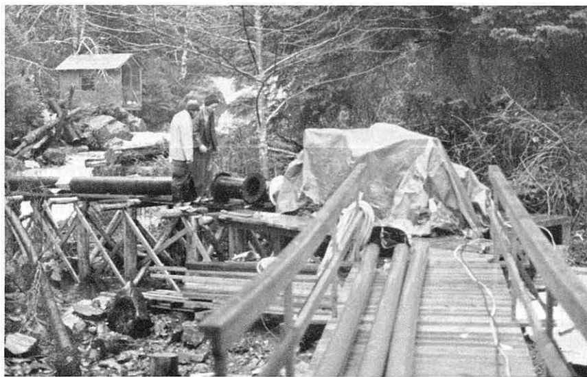
A metal saddle (above) clamps the pipeline. Richard Mathews and an assistant (left) prepare to install the 300 lb. gate valve.
