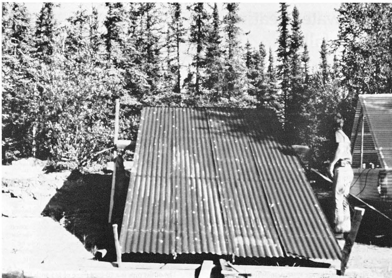
The first solar collector (above) was constructed on the ground.
