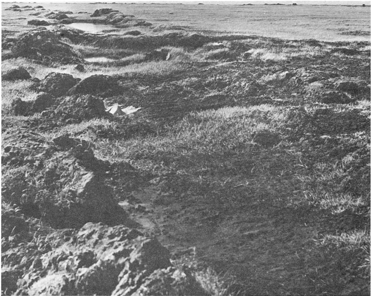
Photo 1: A bladed summer trail with distinct berm of sod and vegetation (Cape Simpson).
