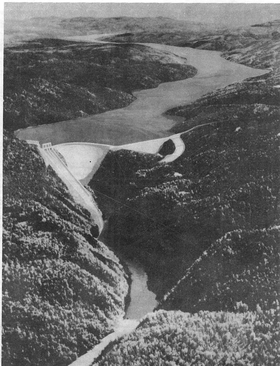
The Watana dam would be an earth-fill structure 885 feet high, 4100 feet long, with an installed capacity of 1020 MW. The Devil Canyon dam would be a concrete arch dam 645 feet high, about 1500 feet long at the crest, with an installed capacity of 600 MW. The Watana dam would create a reservoir 48 miles long; Devil Canyon a reservoir 26 miles long.
