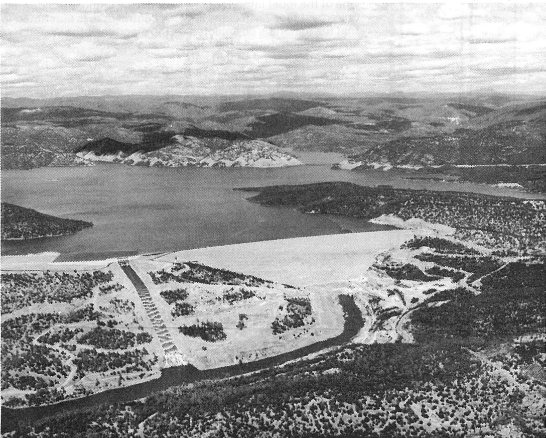
The design of the Oroville dam in California has been suggested as an appropriate model for preliminary design of the Watana dam. It is an earthfill dam like Watana is proposed to be, is in a seismic area, and is of a similar height (Oroville is 770 feet, Watana is proposed to be 880 feet).
