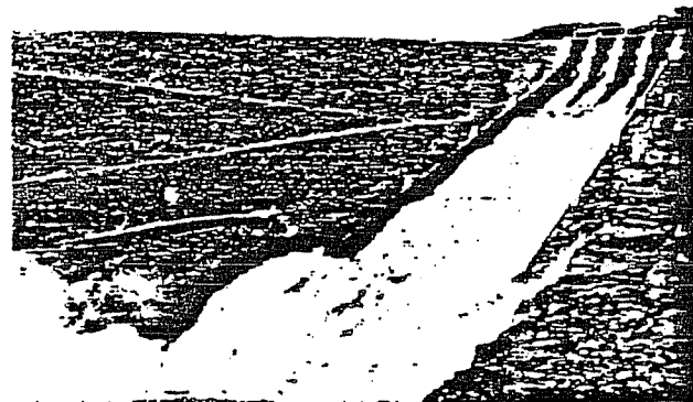
Foz do Areia dam spillway discharging 2500 m³/s.
