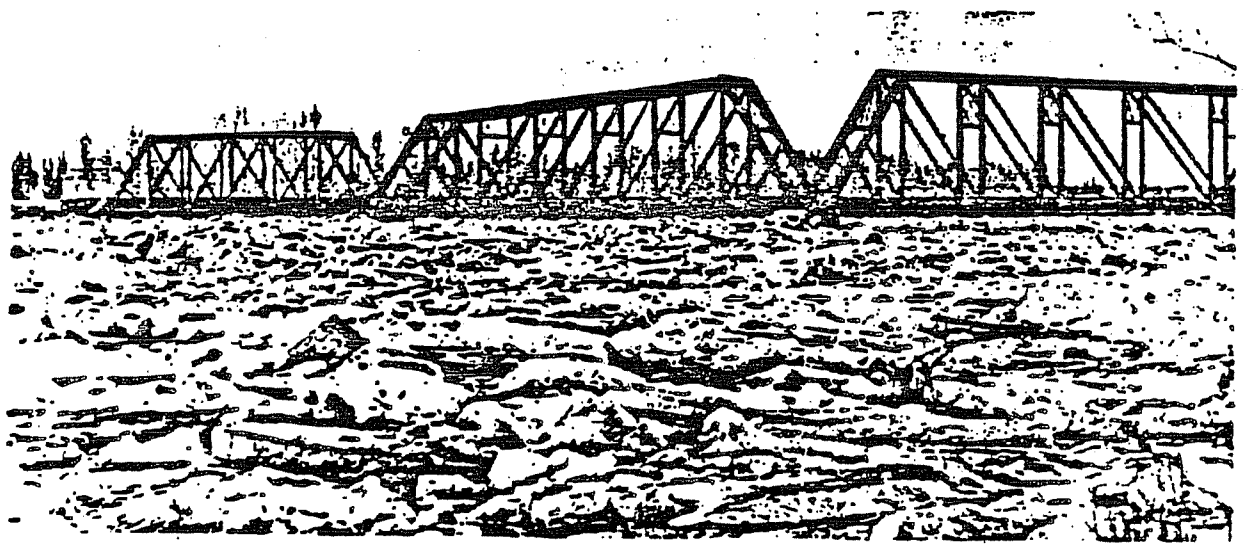
Figure 23 McLeod River - ice jam at railway bridge. Water level is 6 - 8 m above normal.
