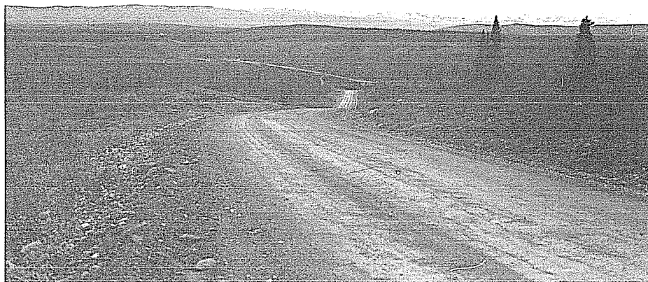
PHOTO 8.D.3 DENALI HIGHWAY (LOOKING SOUTHEAST) NEAR PROPOSED ACCESS ROAD JUNCTION. THIS IS A TYPICAL COMPACTED GRAVEL ROAD AND IS SIMILAR TO THE PROPOSED ACCESS ROAD
