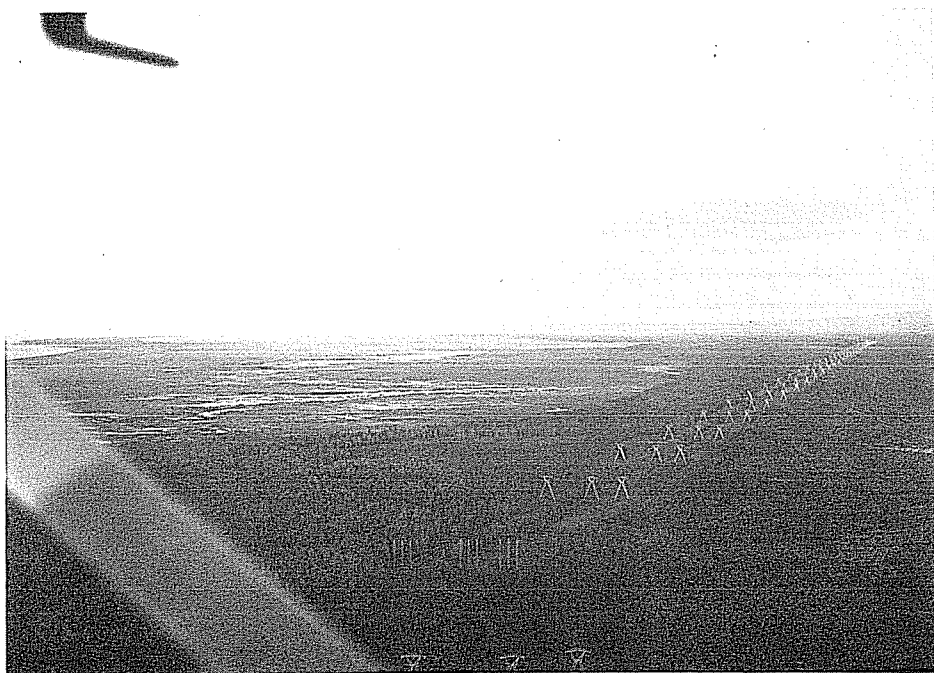
PHOTO 8.D.12 EXISTING TRANSMISSION LINES NORTH SIDE OF COOK INLET - SUSITNA RIVER LOWLANDS. THIS CORRIDOR IS SIMILAR IN SIZE AND TOWER DESIGN TO THE DEVIL CANYON TO GOLD CREEK CORRIDOR. NOTE THE STRAIGHT ALIGNMENT AND RIGID VEGETATION EDGES
