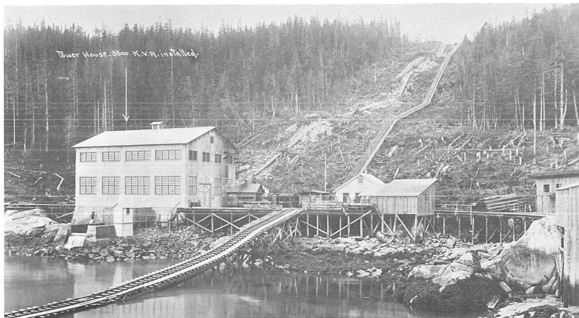
Figure 15. Powerhouse number 1 of the Salmon Creek project was located at tidewater. A small railroad connected this facility to powerhouse number 2 which was located above it.
