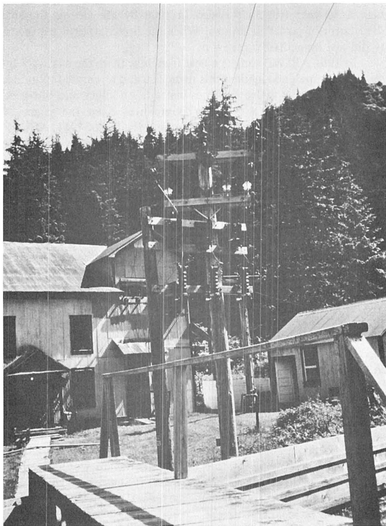
Figure 13. Powerhouse number 2 of the Salmon Creek project looked much the same in 1981 as when it was built in 1914.
