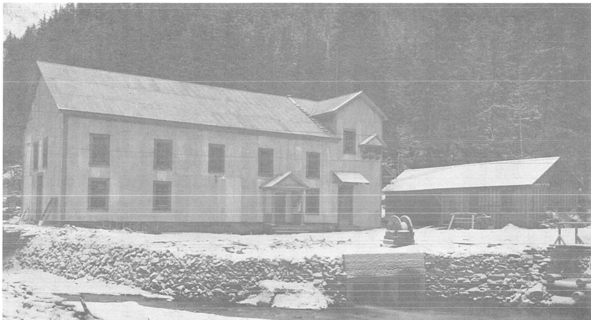
Figure 12. Powerhouse number 2 of the Salmon Creek project near Juneau has been supplying electricity from 1915 to the present day.
