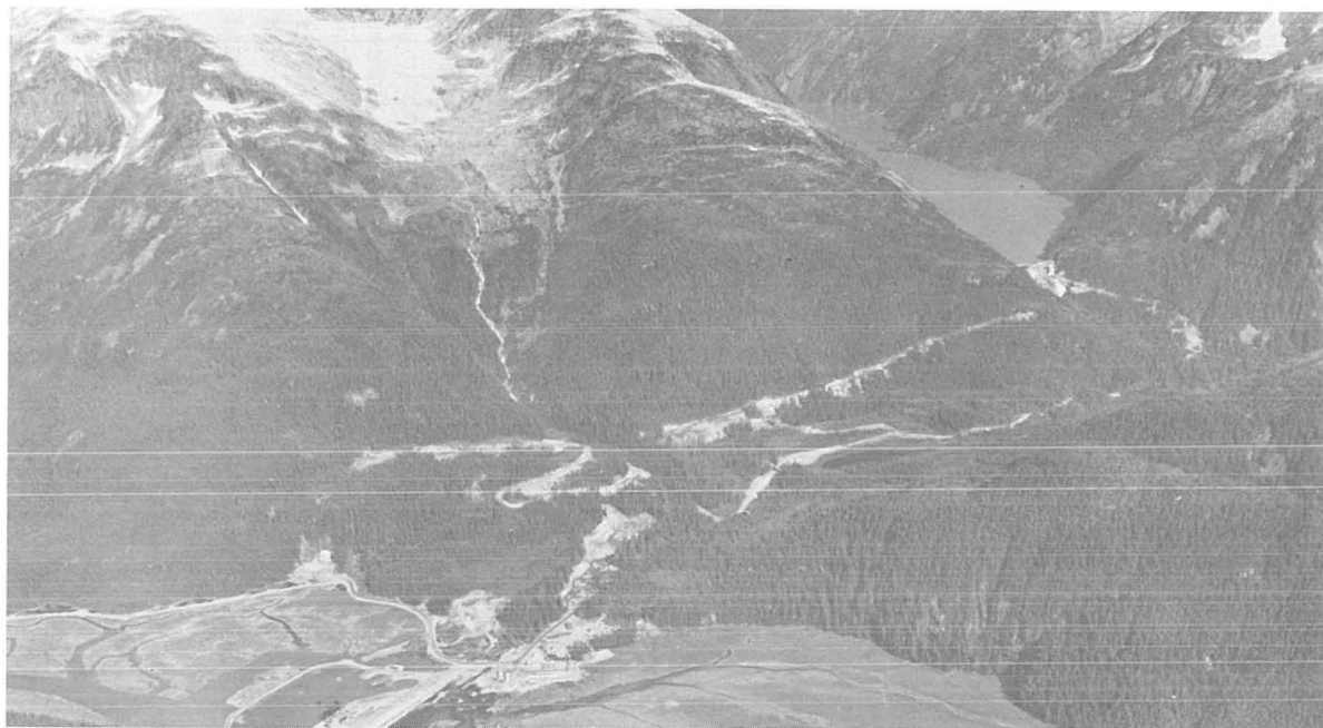
Figure 33. The Long Lake reservoir supplies power to Juneau's Snettisham project.
