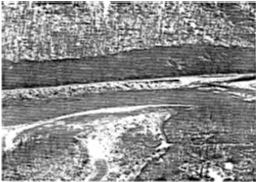
Overflow Channel, River Mile 142.2
