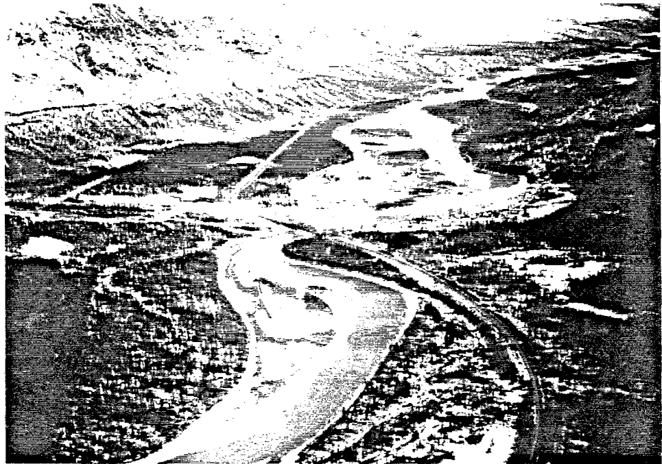
Gold Creek Railroad Bridge, River Mile 136.7
