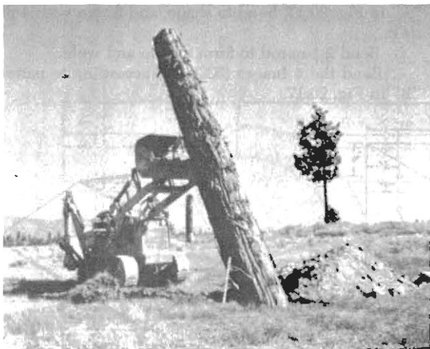
C. Erecting a cedar pole.
