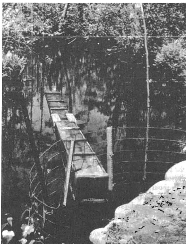
Fig. 20.32. Wire mesh fence to protect culvert from flooding with a “beaver pipe” (H. Nevers, N. Hampshire Fish and Game Department).
