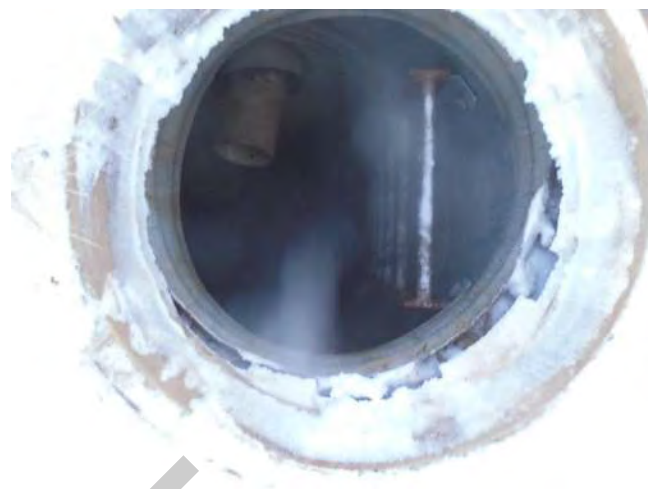
MH14A view from above with PVC inlet in view.
