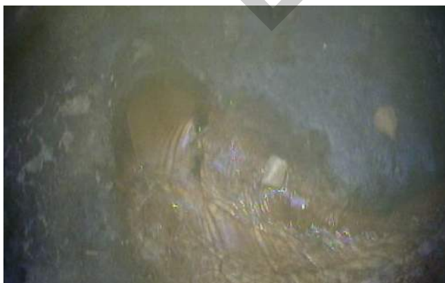
STEP service line into MH1.
