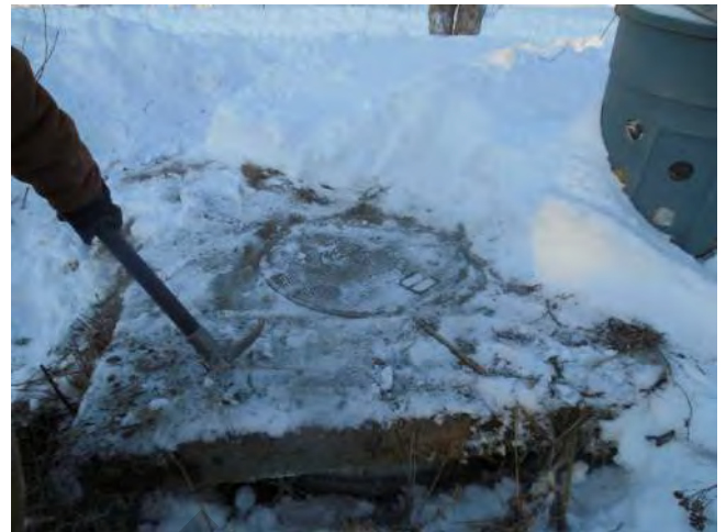
MH3 concrete lit with metal cover.
