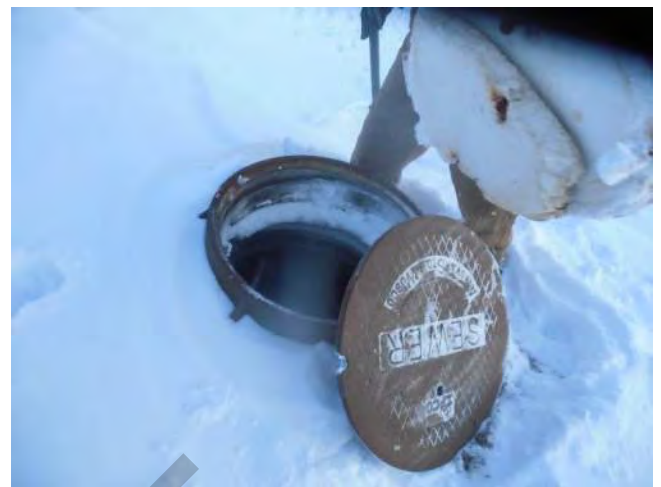
MH14C with lid and insulation plug.
