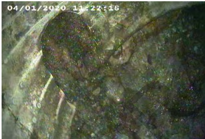
MH3B collapsed pipe or nonexistent pipe with barrel notch.
