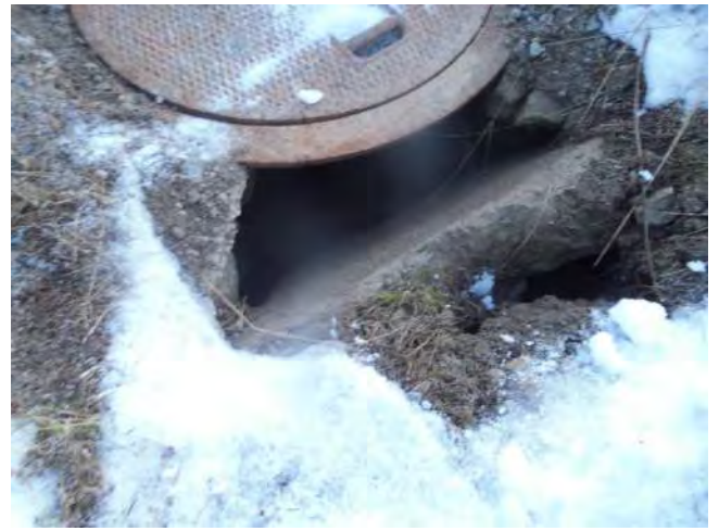
MH11 cement deterioration.
