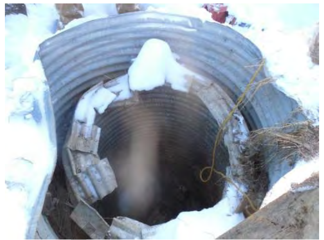
MH14 with 60" Lid and 42" barrel..
