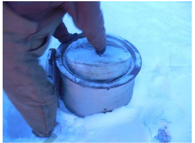
Opening MH14F and removing insulation plug.
