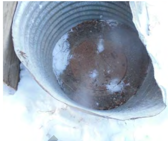
Insulation plug in MH1.
