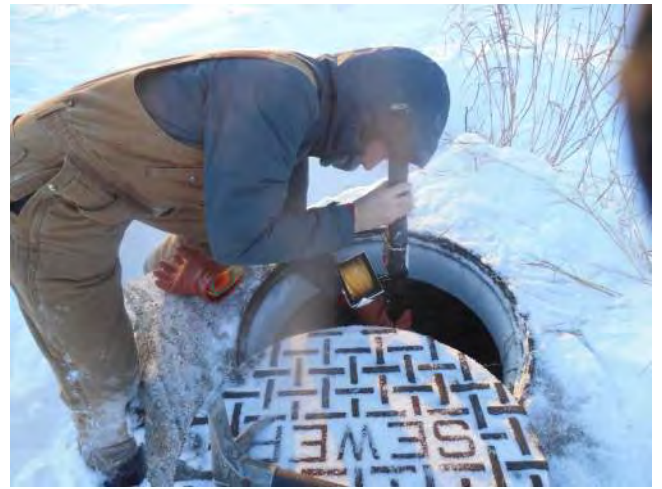
Using camera in MH8.
