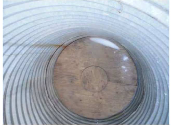
MH7C insulation plug.
