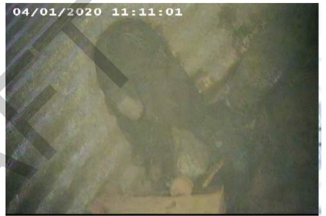
MH3C collapsed pipe or nonexistent pipe with barrel notch..
