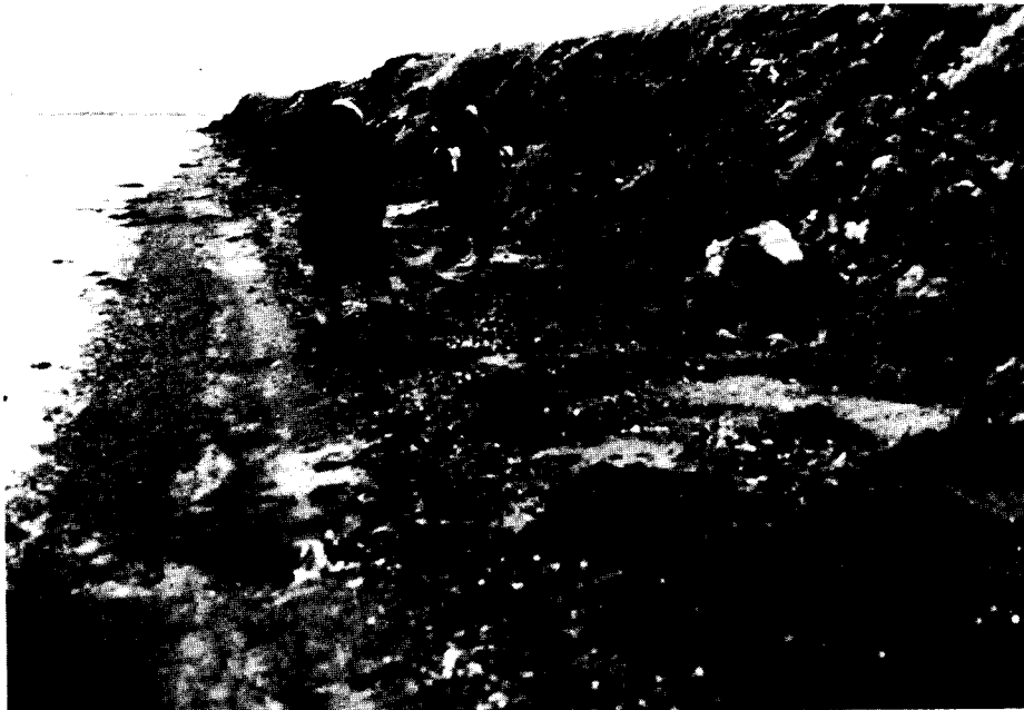
Figure 4-10. Rapidly retreating low tundra cliff in Kugrua Bay. Note the narrowness of the beach and the reworked peat blocks on the beach surface.
