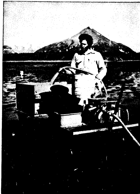
Photograph 12. Biologist using the Homelite pump mounted on the wagon to wash the subsample which is inside the box.
