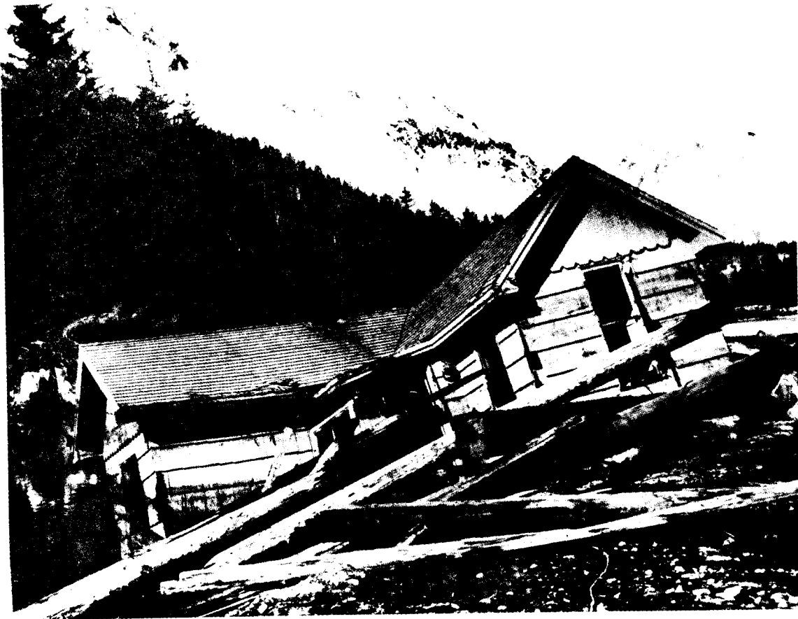
Figure 5. Seward (Alaska) residence severely damaged by tsunami of March 27, 1964. The tsunami caused heavy damage at many other port towns in southern Alaska.
