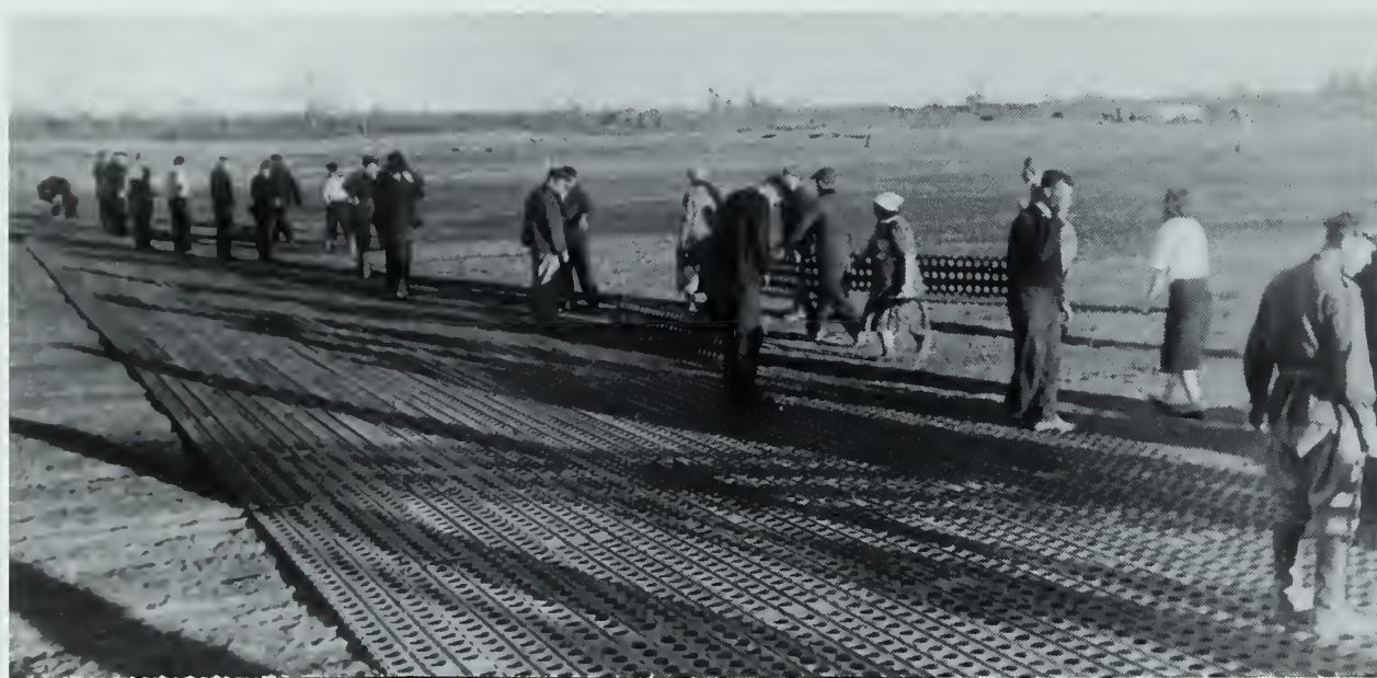
The laying of metal mats (pierced steel planking – PSP) for takeoff and landing strips (VPP) in Markovo, August 1943.
