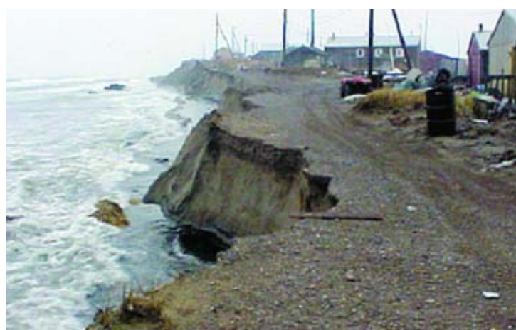
Figure 6. Two photos of a coastal road in the community of Shishmaref. The first photo was taken around 12:30 pm on October 8, 2002 while the second photo was taken some two hours later. During that period the shoreline had eroded through the road (notice the tire tracks).
