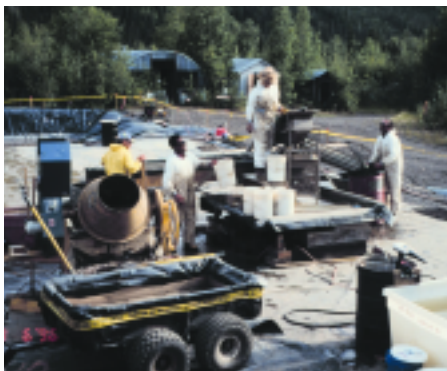
Overview of soil-washing process to remove mercury from soil.
