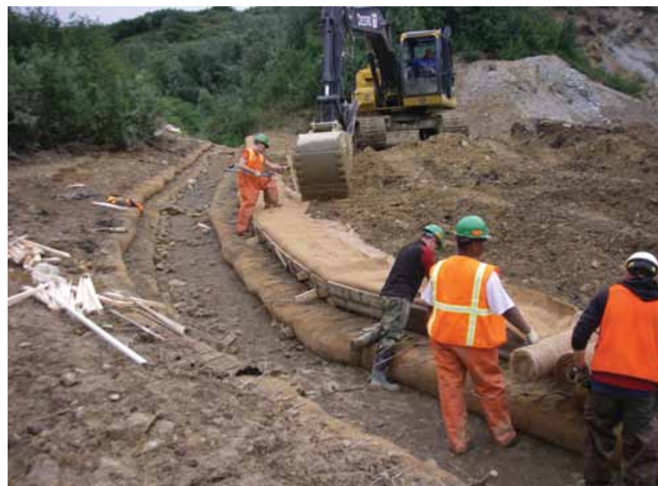
Figure 5. Construction of FES stream banks at Slate Creek.
