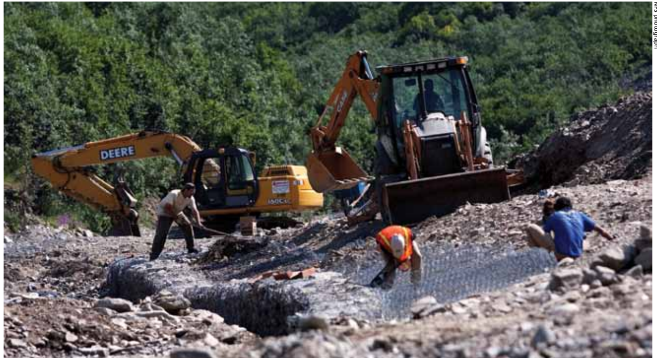
Figure 7. Field crews assemble bank stabilization structures.
