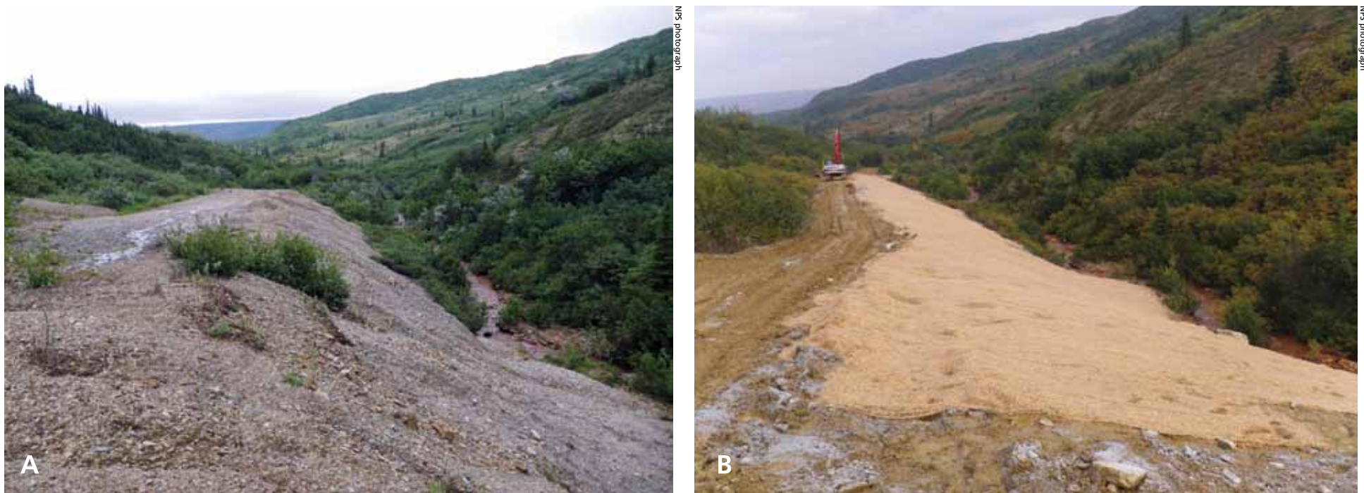
Figure 6a, 6b. View of extended tailings pile showing pre-construction conditions (left) and post-construction slope treatment and erosion blanket installation.
