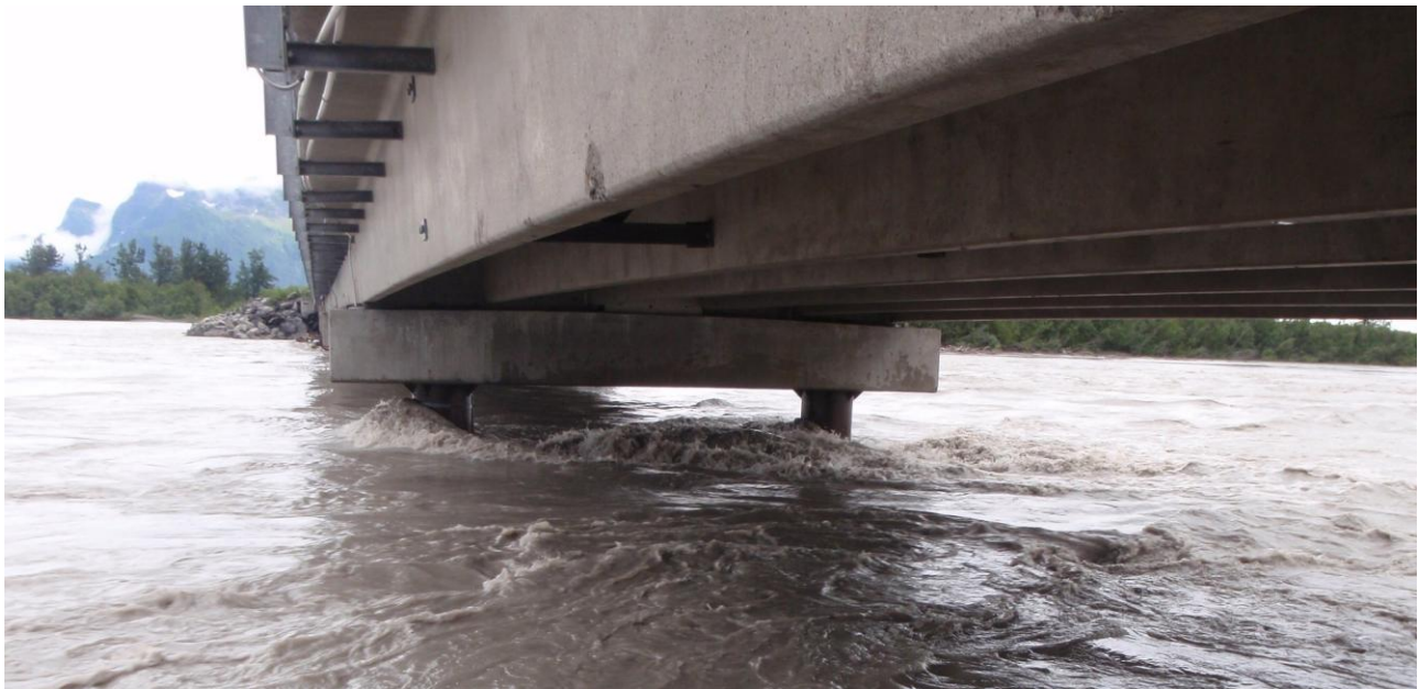
Figure 8. Active Scour on Bridge #339, Copper River Highway
