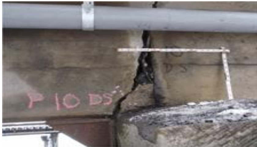
Figure 6. Deteriorating Concrete Trail River Bridge
