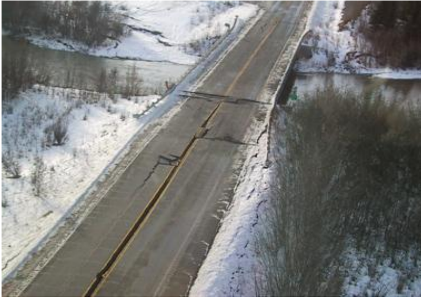
Figure 9: Earthquake Damage on the Richardson Highway
