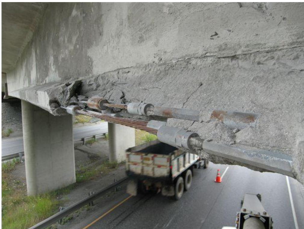
Figure 13. Highway Overpass Damaged by a Vehicle Collision
