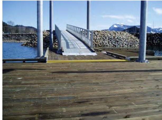
Figure 19. Hoonah Seaplane Float Ramp
