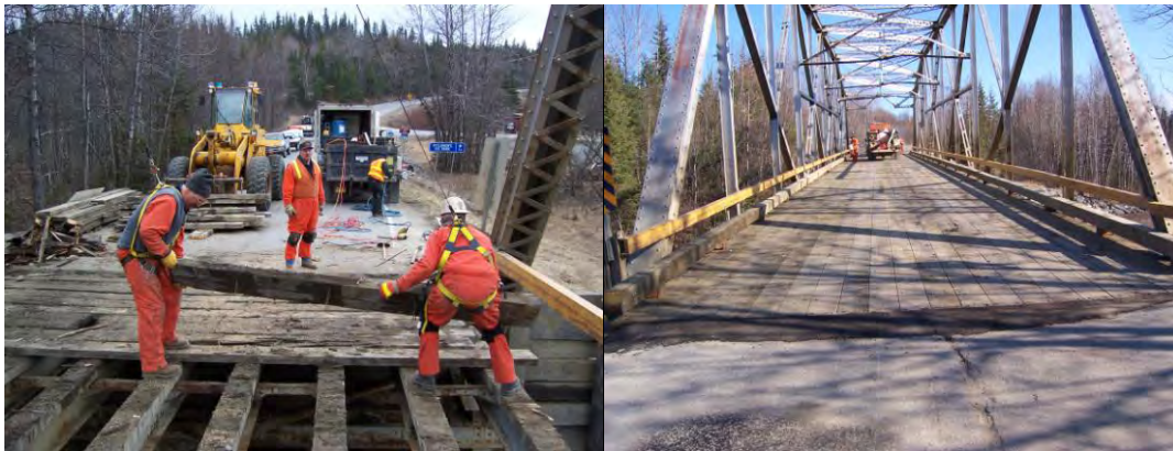
Figure 7. Re-Decking the Anchor River Bridge
