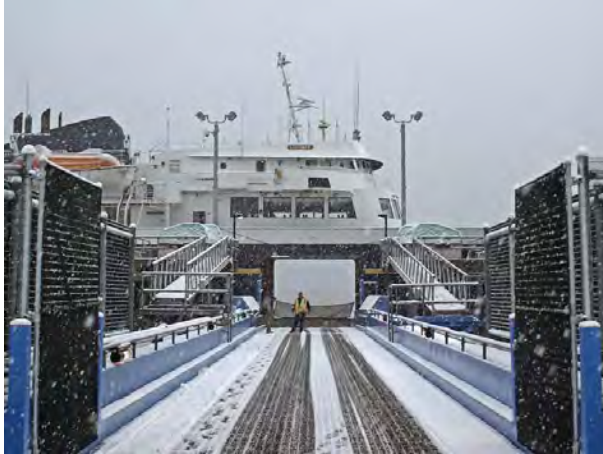
Figure 18. Ferry Terminal Ramp
