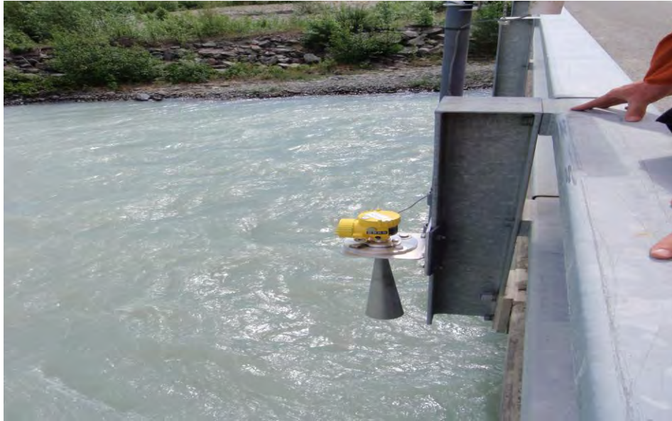
Figure 8. Active Scour Monitoring on the Tonsina River
