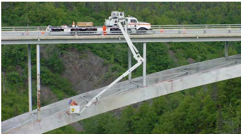
Figure 12. Bridge Inspection at Hurricane Gulch
