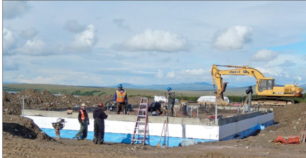
In Golovin, the new water treatment facility is being constructed on higher ground out of the flood zone.
