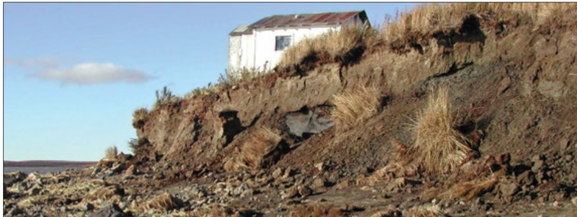
A St. Michael house threatened by erosion. Photo courtesy of Michelle Snowball.
