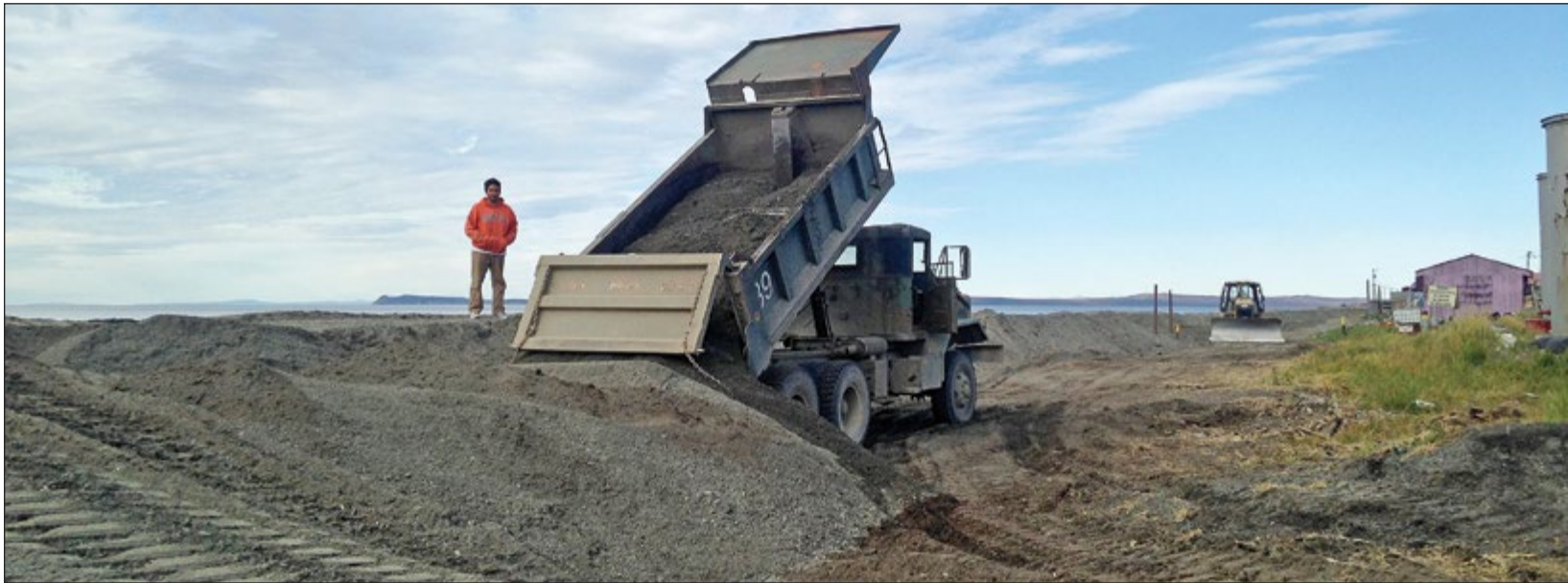
Workers build an earthen berm to help prevent flooding. Photo courtesy of Terry Johnson.
