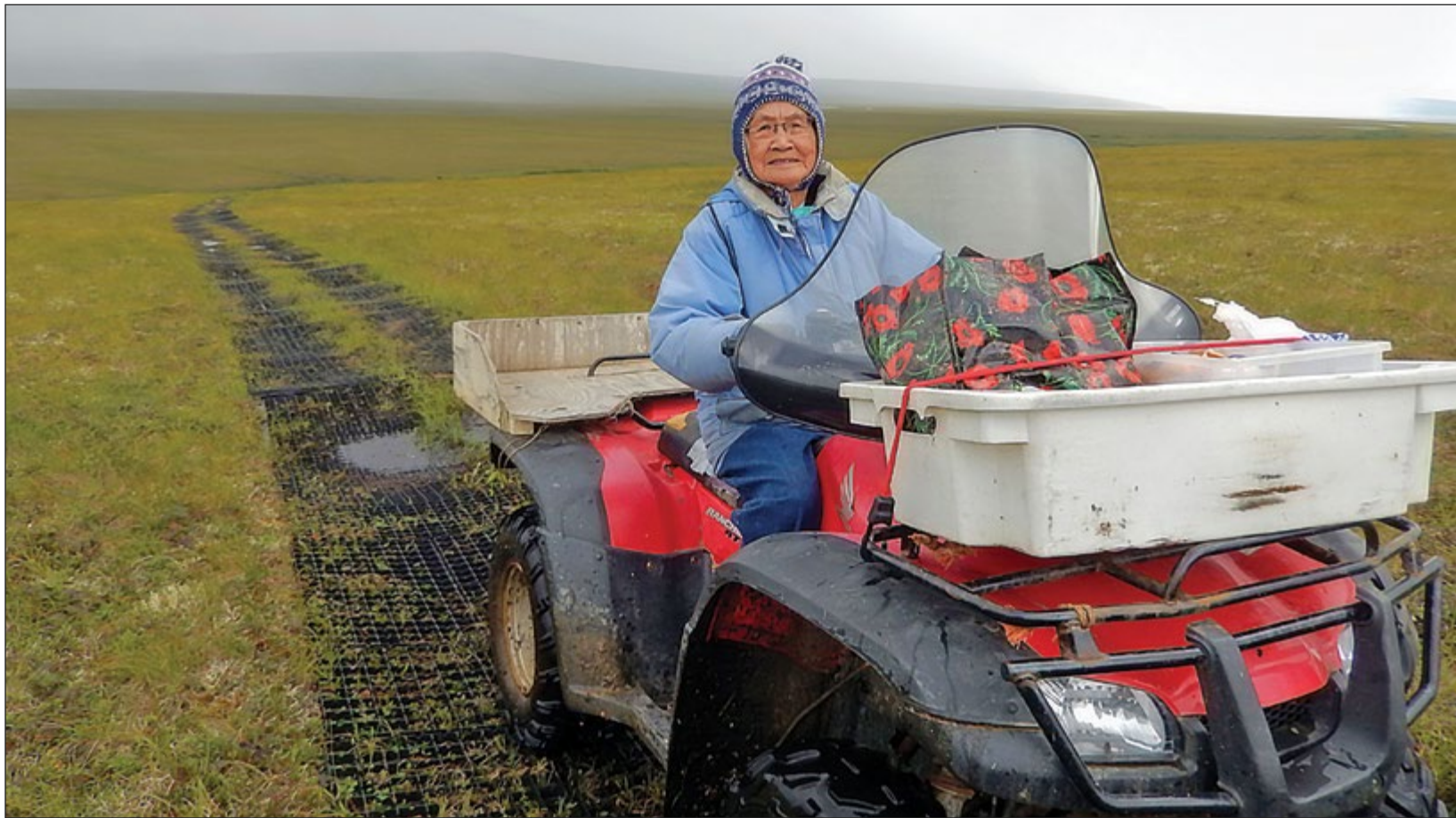
Florence Doyle of Golovin rides her ATV over the geotextile road installed to protect vegetation and prevent thawing.
