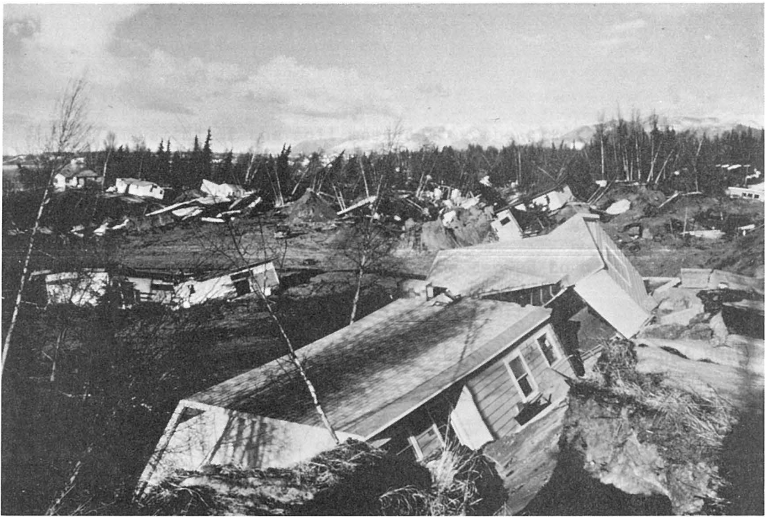
A study conducted by the Engineering Geology Evaluation Group in Anchorage reveals the extent of movement of some of the houses in the slide area. Fig. 4, prepared by this group, shows the initial and final positions of houses as determined by surveys before and after the earthquake. It may be seen that some of the houses moved laterally about
